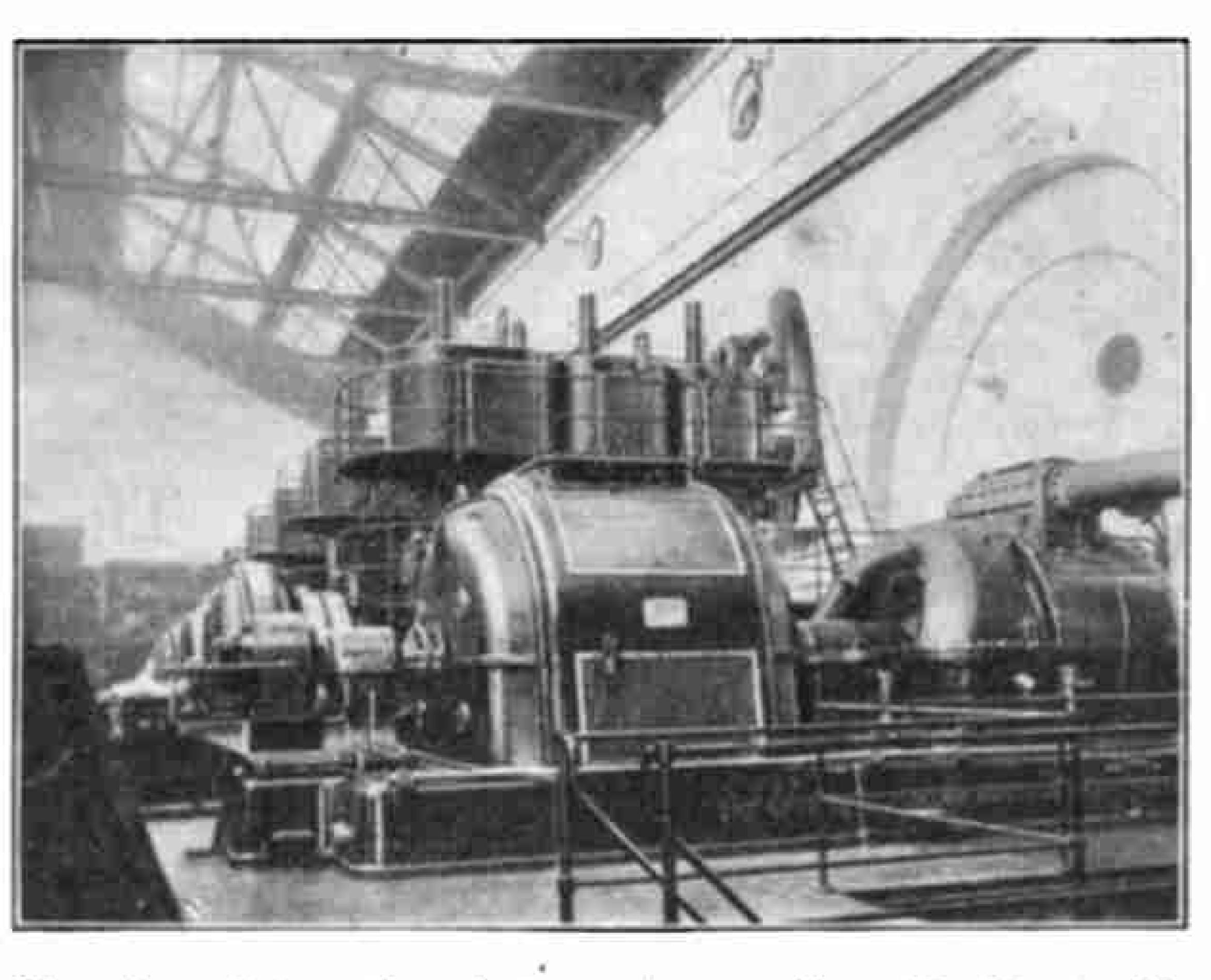
The above interesting photograph (contributed by Master Alan Russell, et Market Rasen), illustrates a line of alternating current dynamos in the Summer Lane Electric Generating Sub-Station at Birmingham. The dynamos are driven by Belliss Triple Expansion engines and the station is mainly used for supplying current to the trams in the city.
