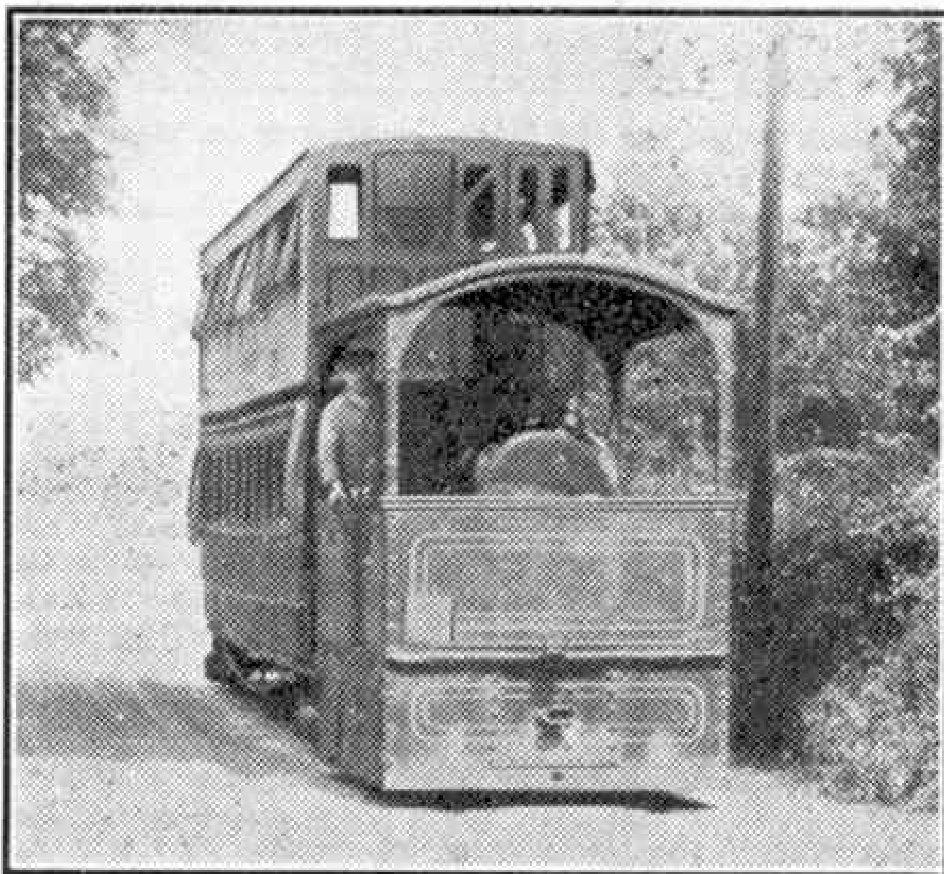
Steam tram that ran on the Wolverton and Stony Stratford Tramway. Photograph by E. Instone, New Bradwell.
