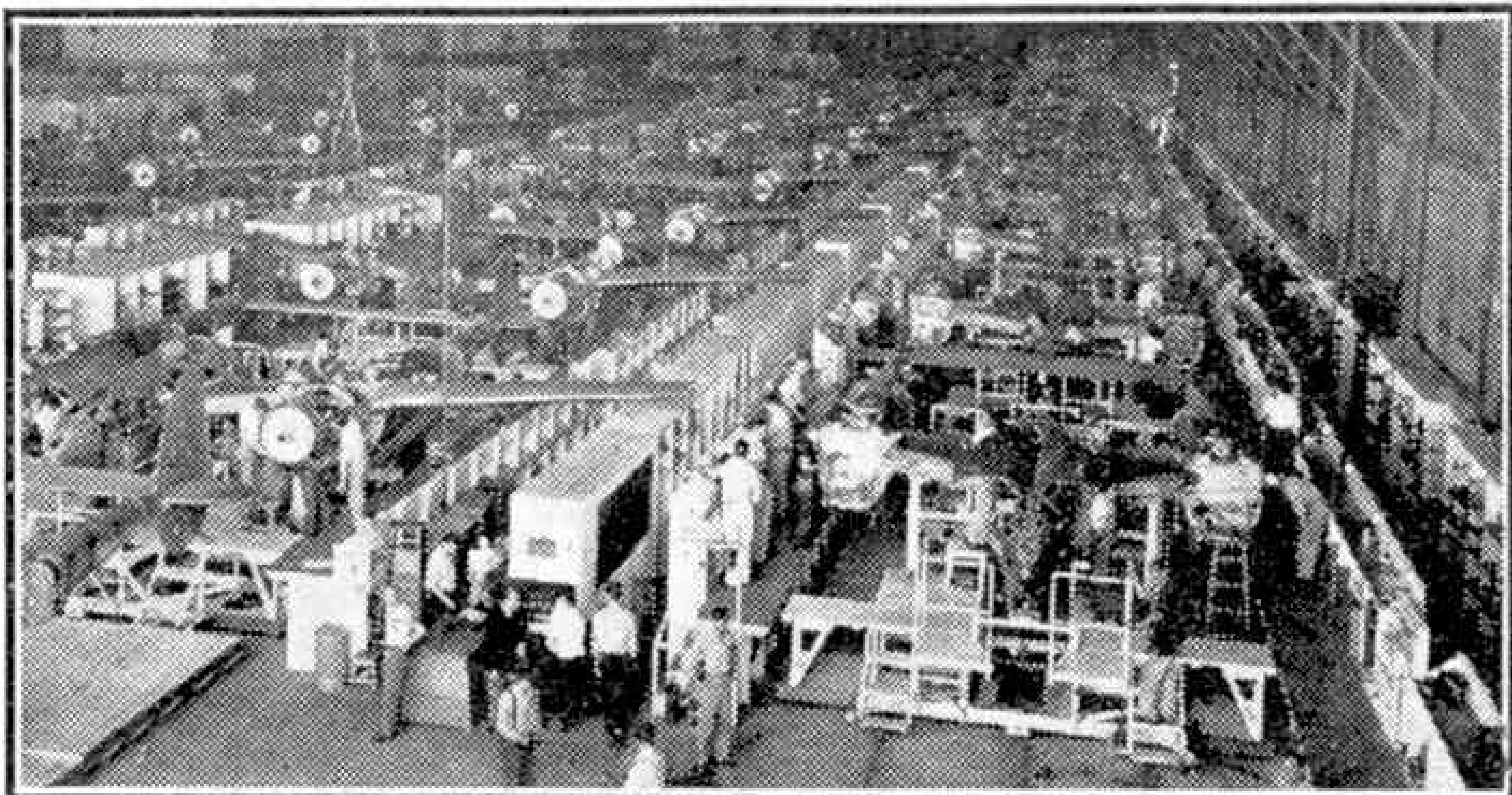
Lockheed P-38 "Lightning" fighters on the new "three abreast" mechanised conveyor lines in the huge Final Assembly hangar at Burbank, California.
