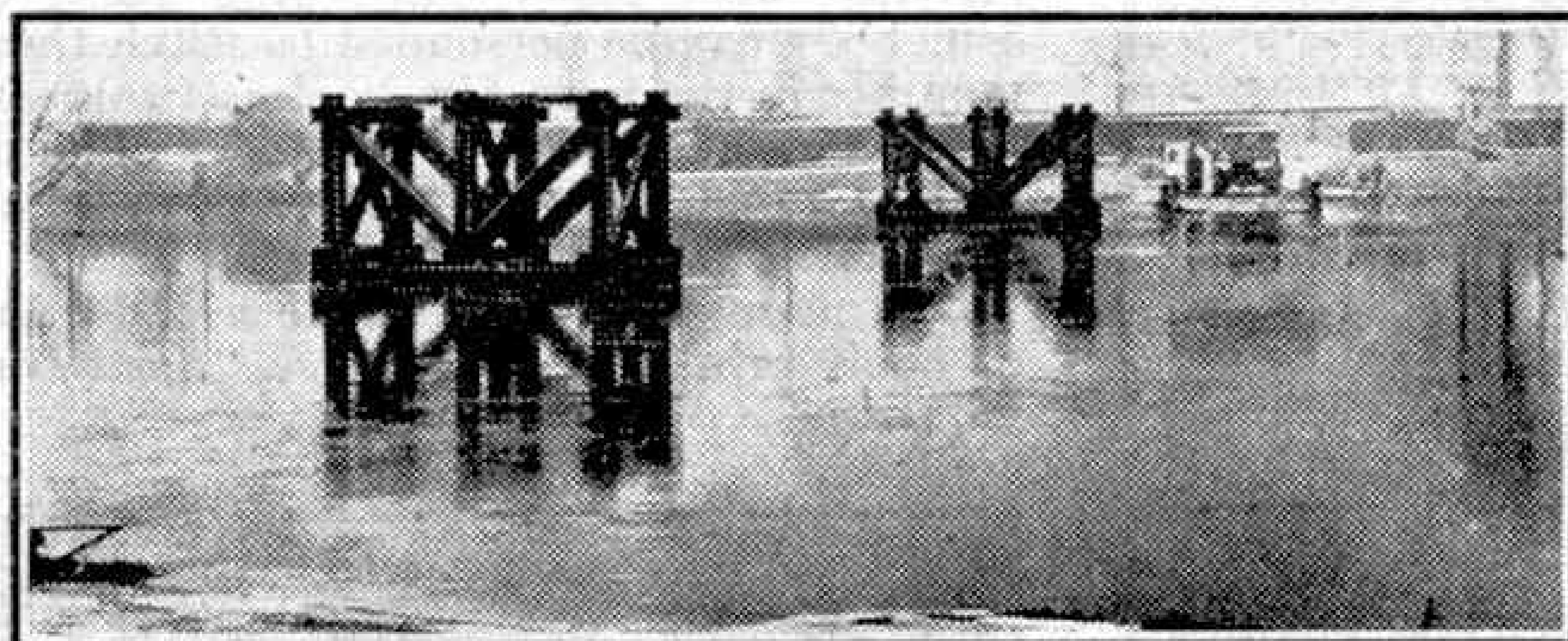
The wooden piers erected; each of six piles 14 in. by 14 in. suitably braced.
