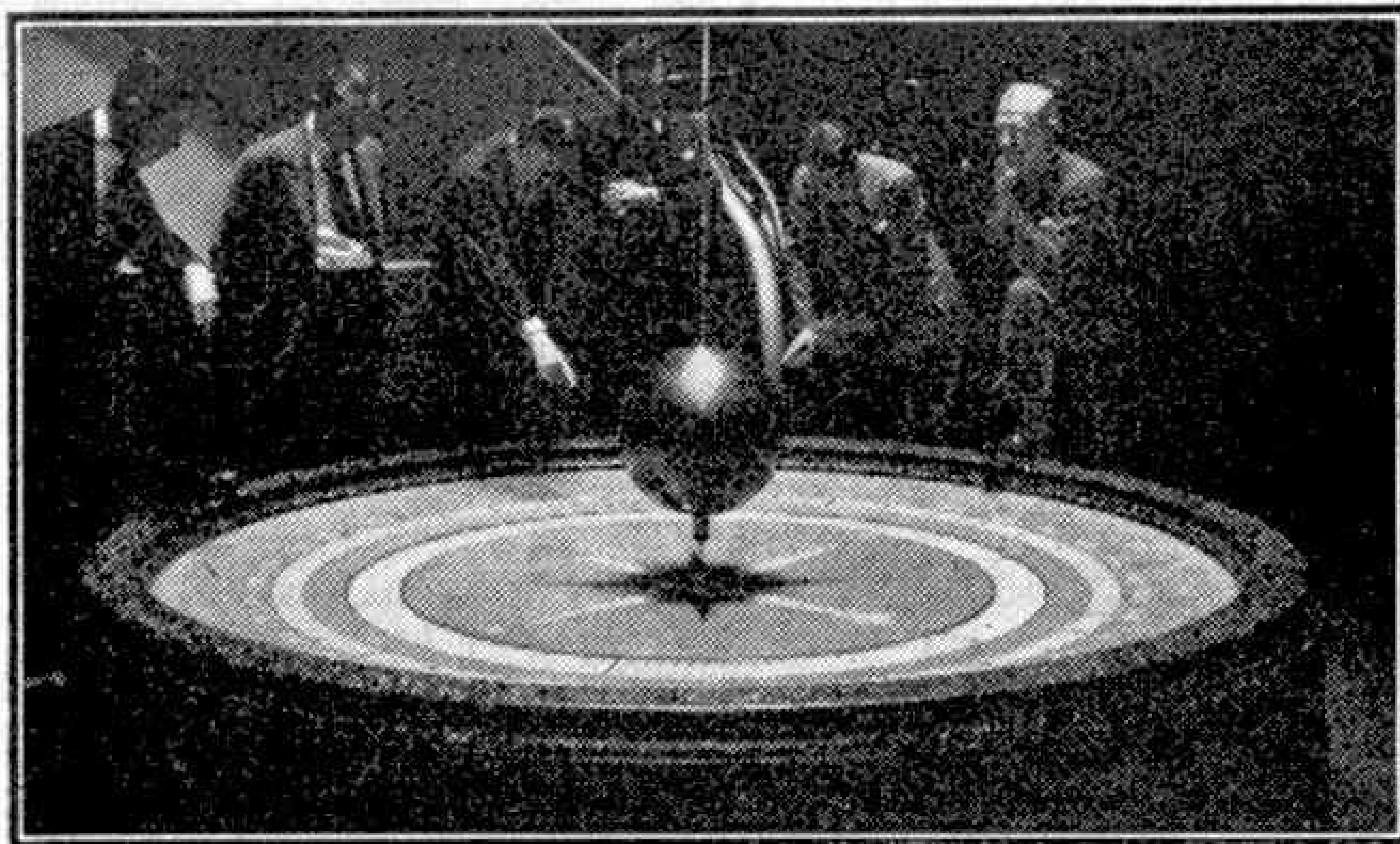
Proving that the Earth turns. The giant pendulum, 65 ft. in length, in the Hall of the Chicago Museum of Science and Industry, that seems to alter in direction as it swings to and fro.
