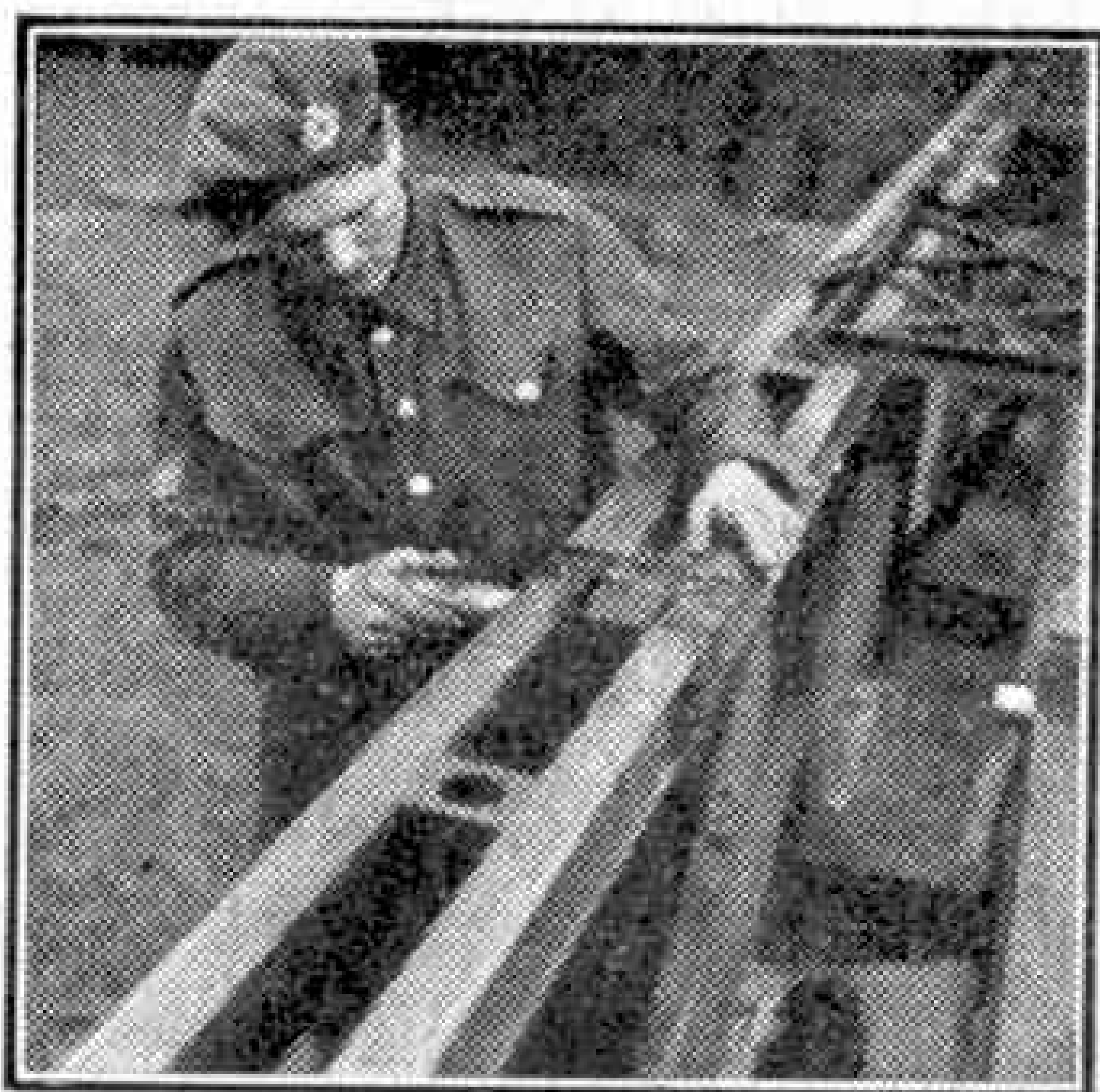
Joints between the sections are secured by driving in 2 in. pins.
