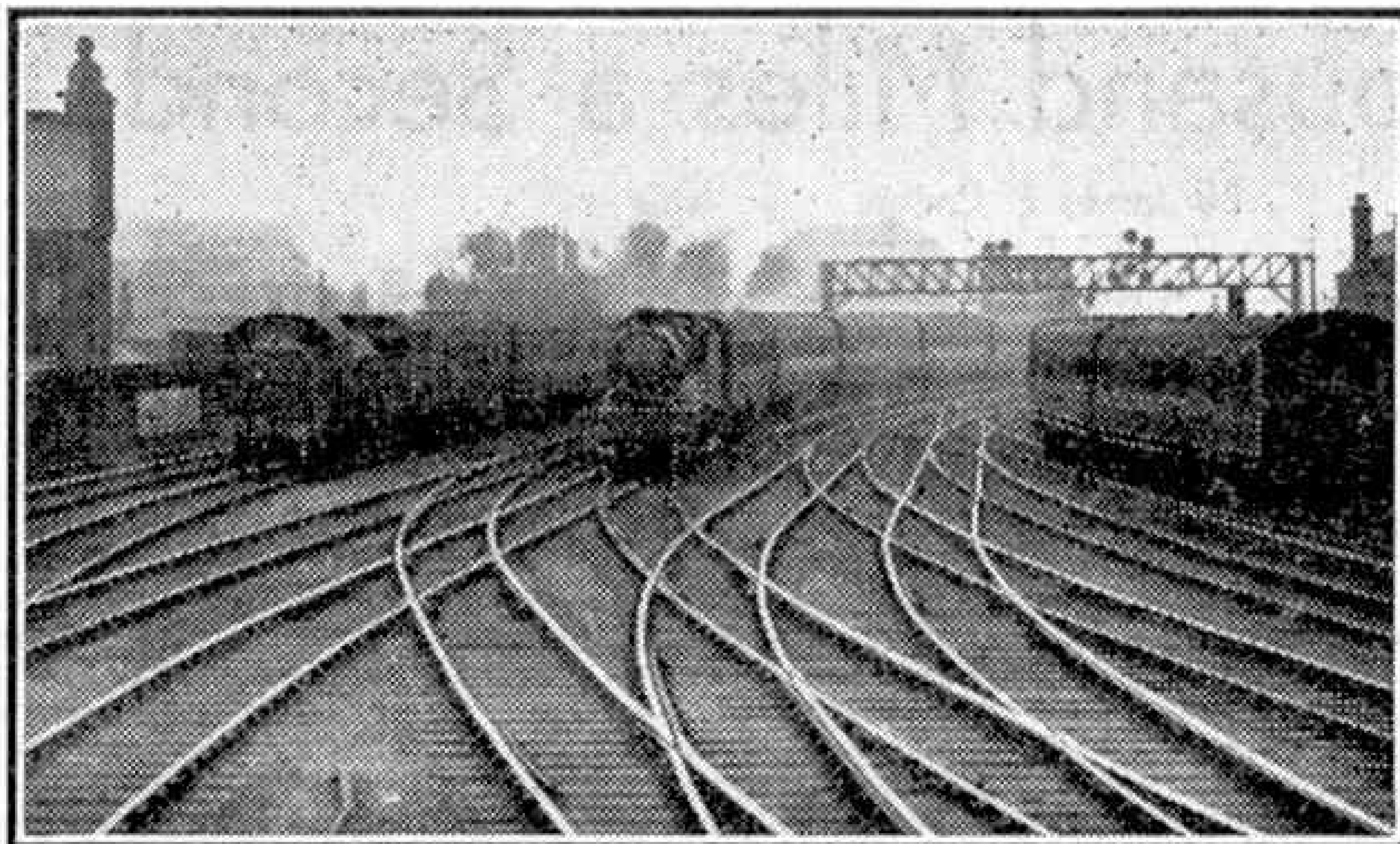
Curves, points and crossings at the approach to a large station. Photograph by courtesy of the L.M.S.R.
