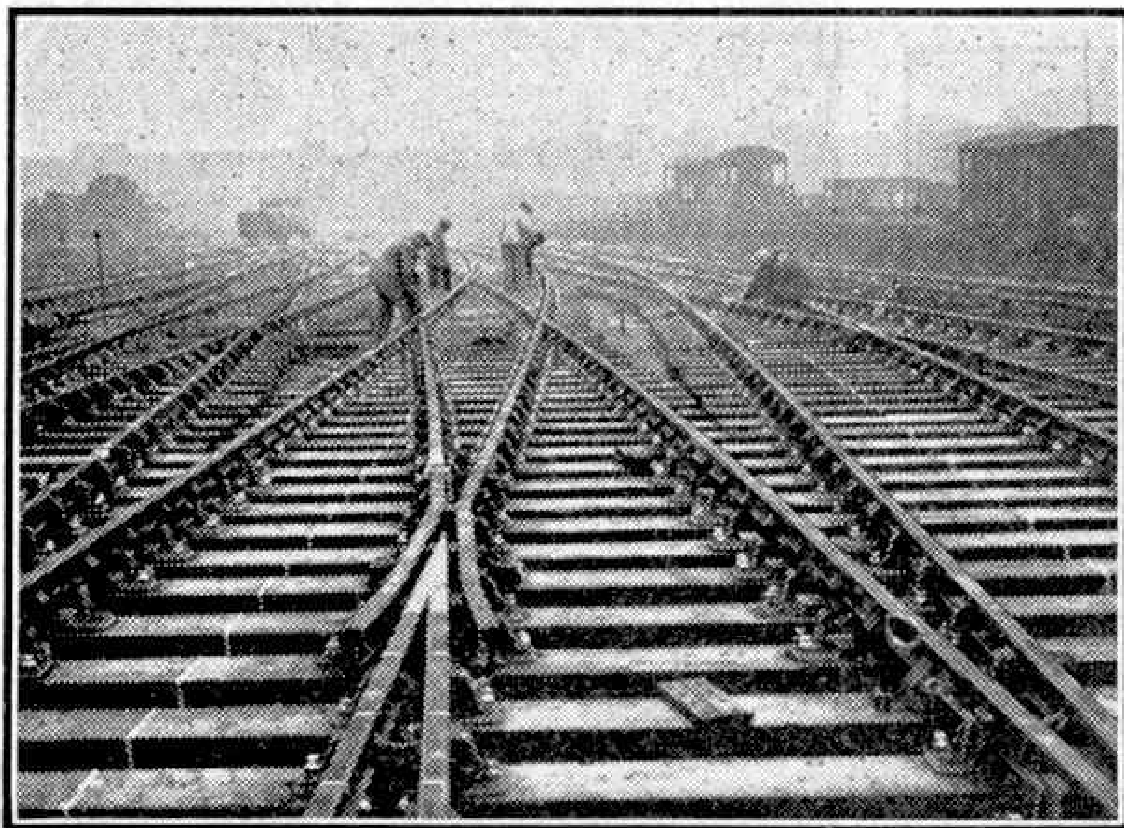
Relaying a junction; "V-crossing" in foreground. This photograph and the lower one on the opposite page are reproduced by courtesy of the Southern Railway.
