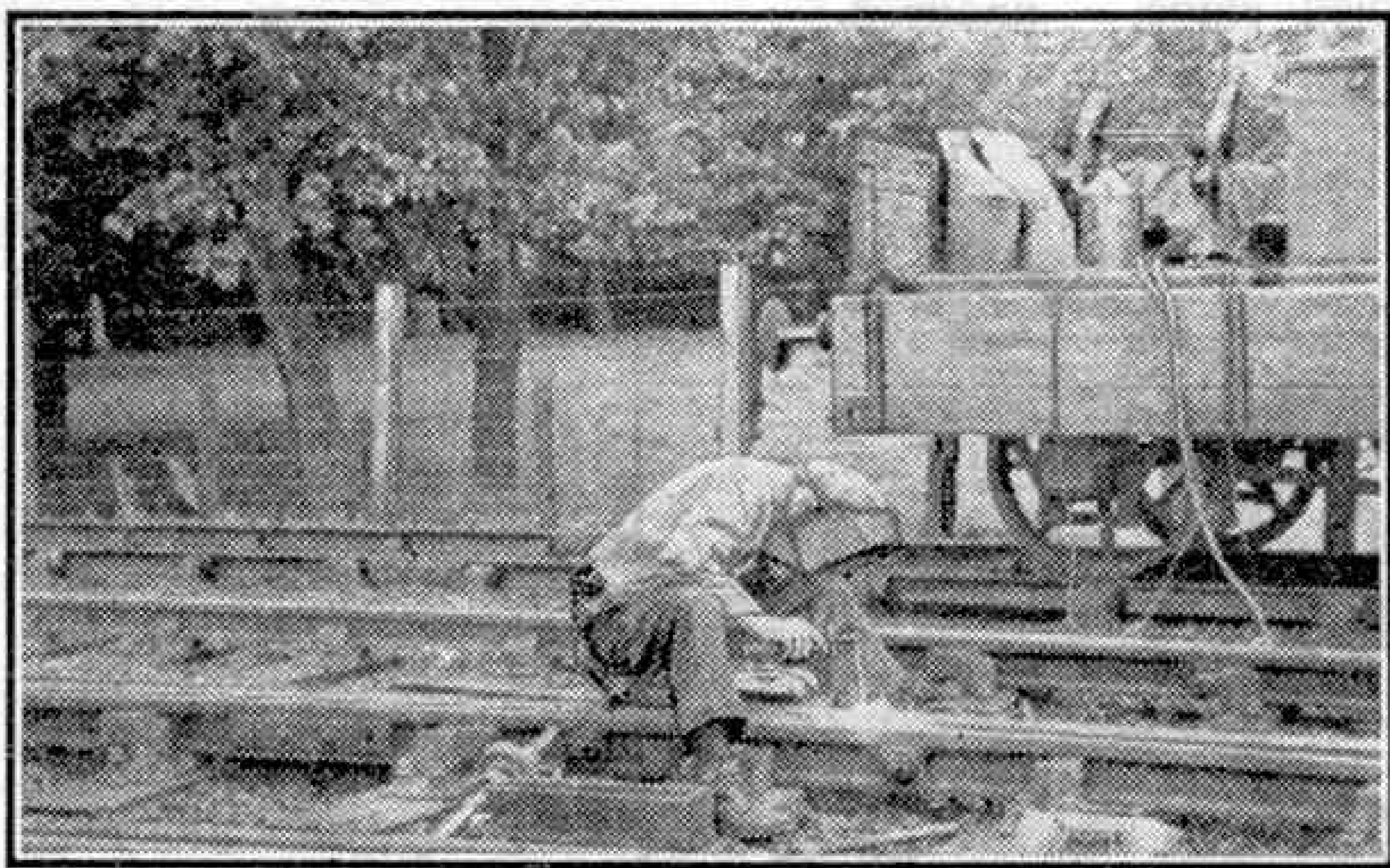
A permanent way welder at work, showing the specially fitted wagon with all the gear.
