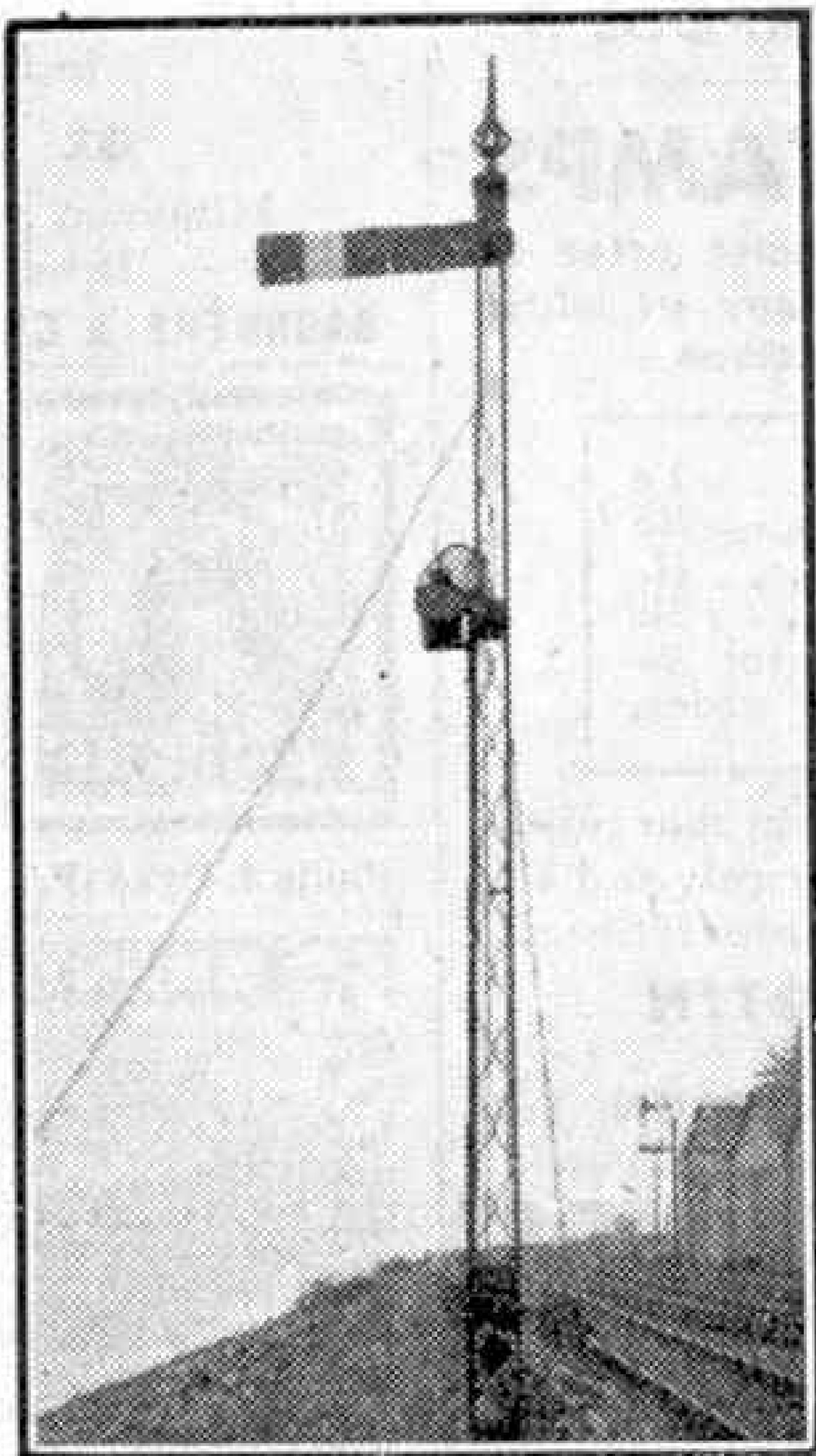
An old type Furness Railway signal at Greenodd, with the lamp and spectacle mounted lower than the arm. Photograph by W. S. Garth, Luton.
