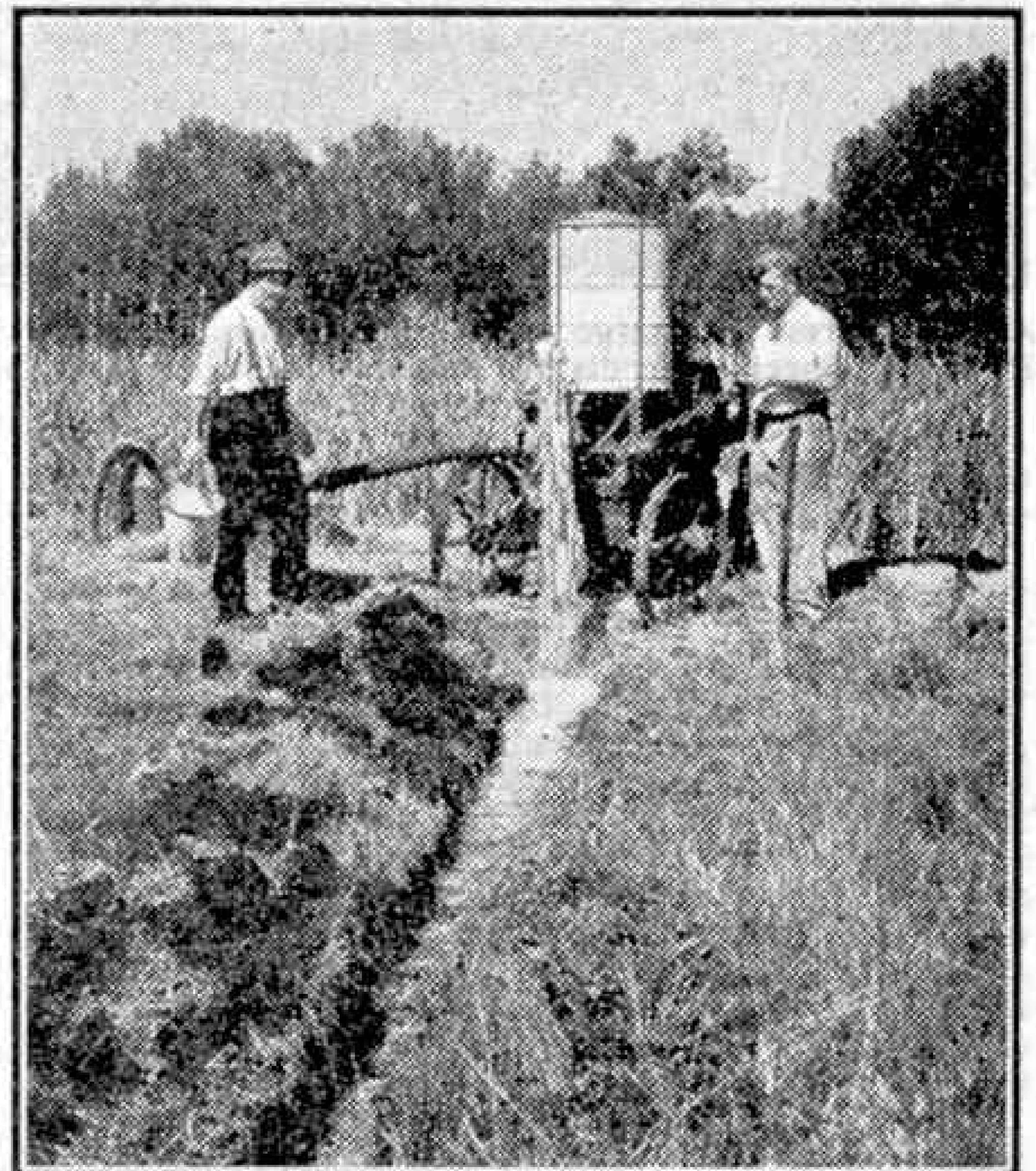
A 5 h.p. diesel engine pump removes water from the pit to a drainage ditch.
