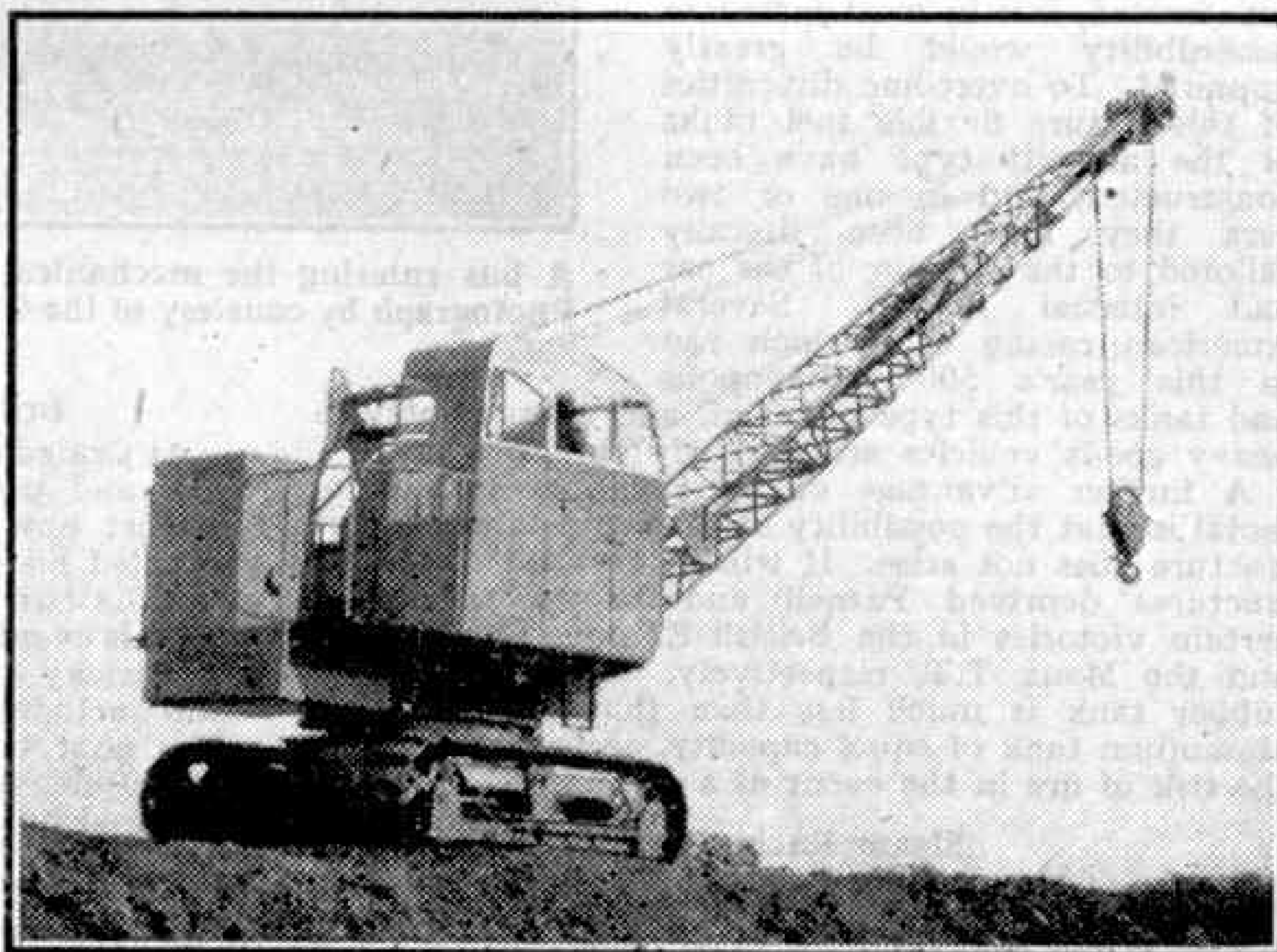
The Jones "Super 40" mounted on crawler tracks.
