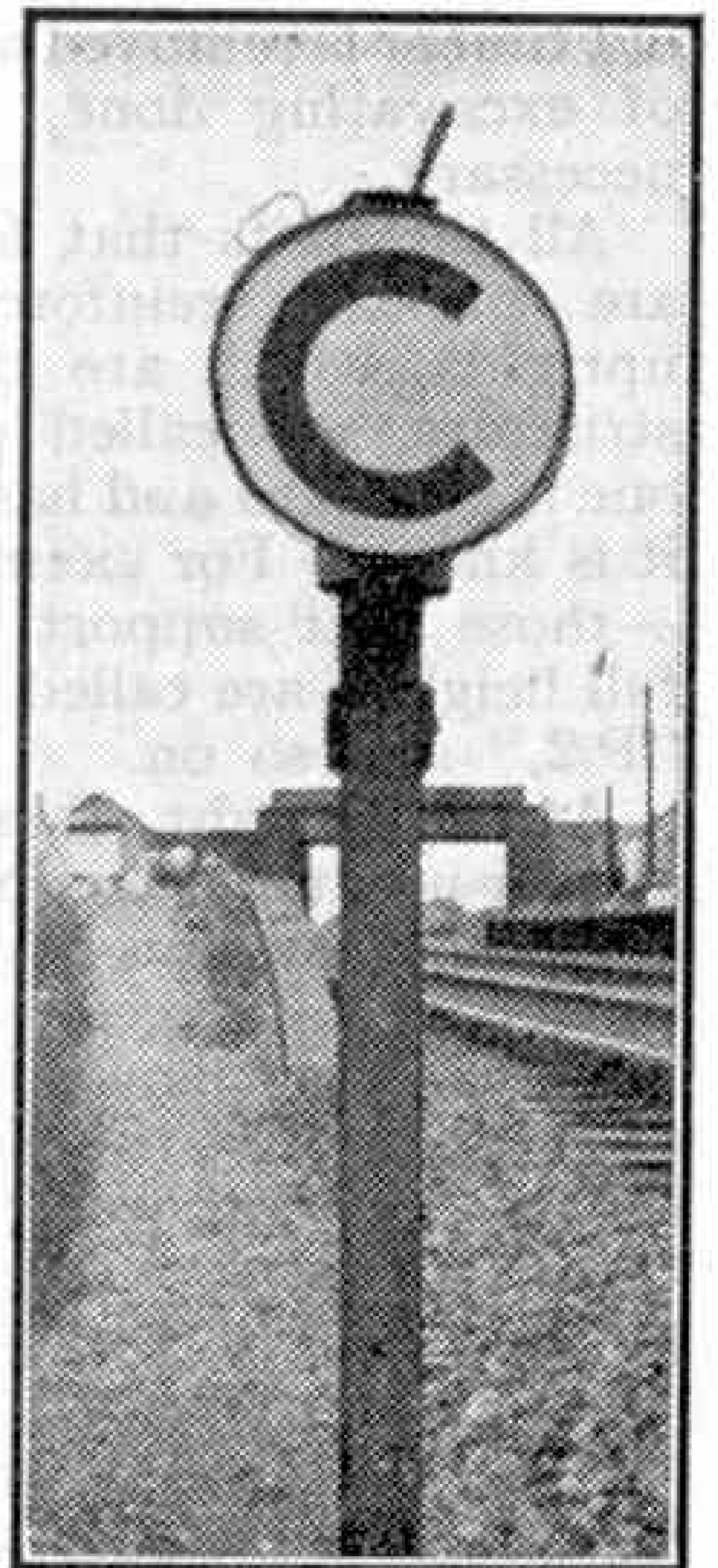
The "C" sign shows where the slack begins.
