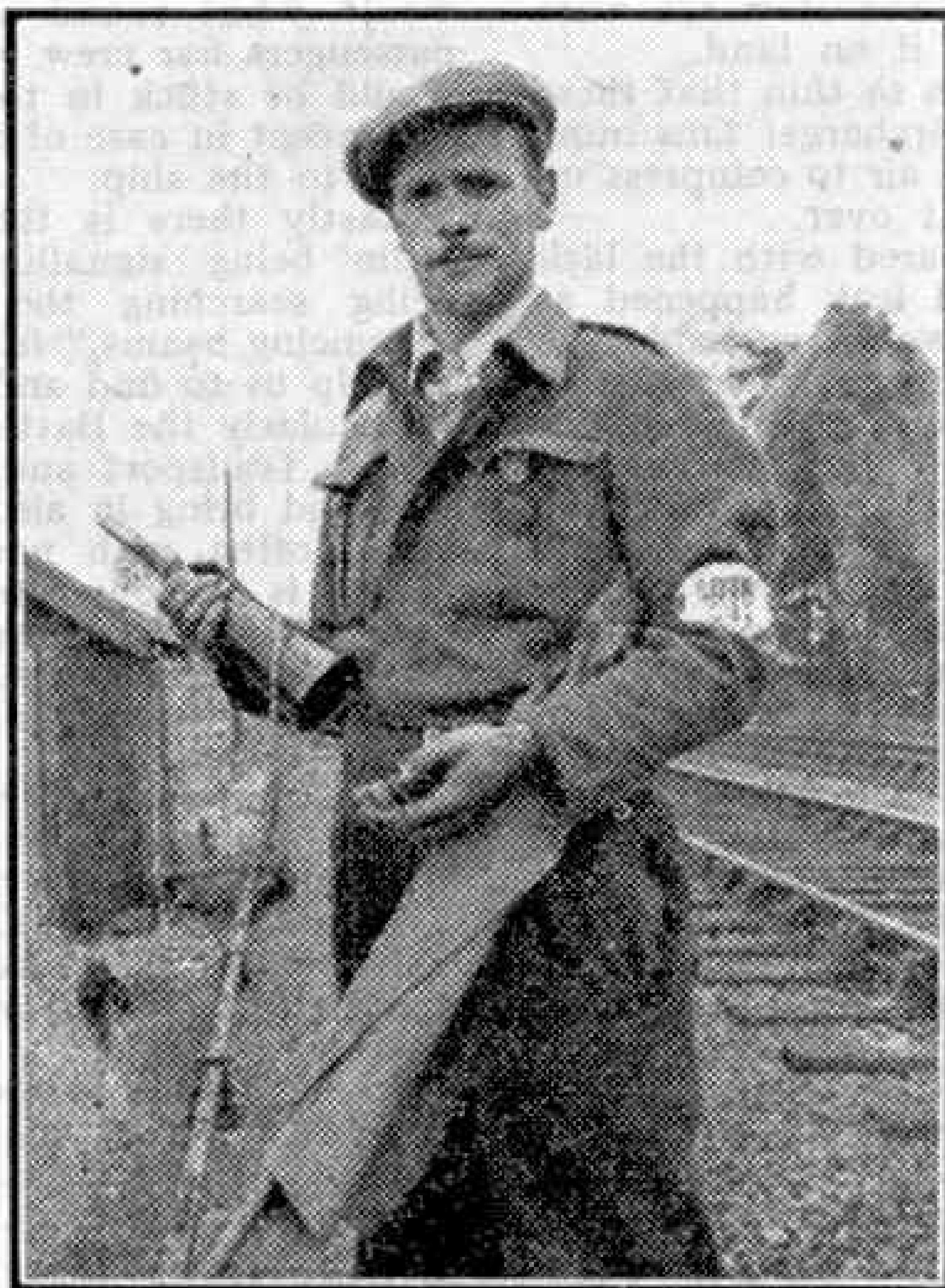
The look-out man with his warning equipment, and distinctive armlet. He carries red and green flags, detonators and a horn or whistle.
