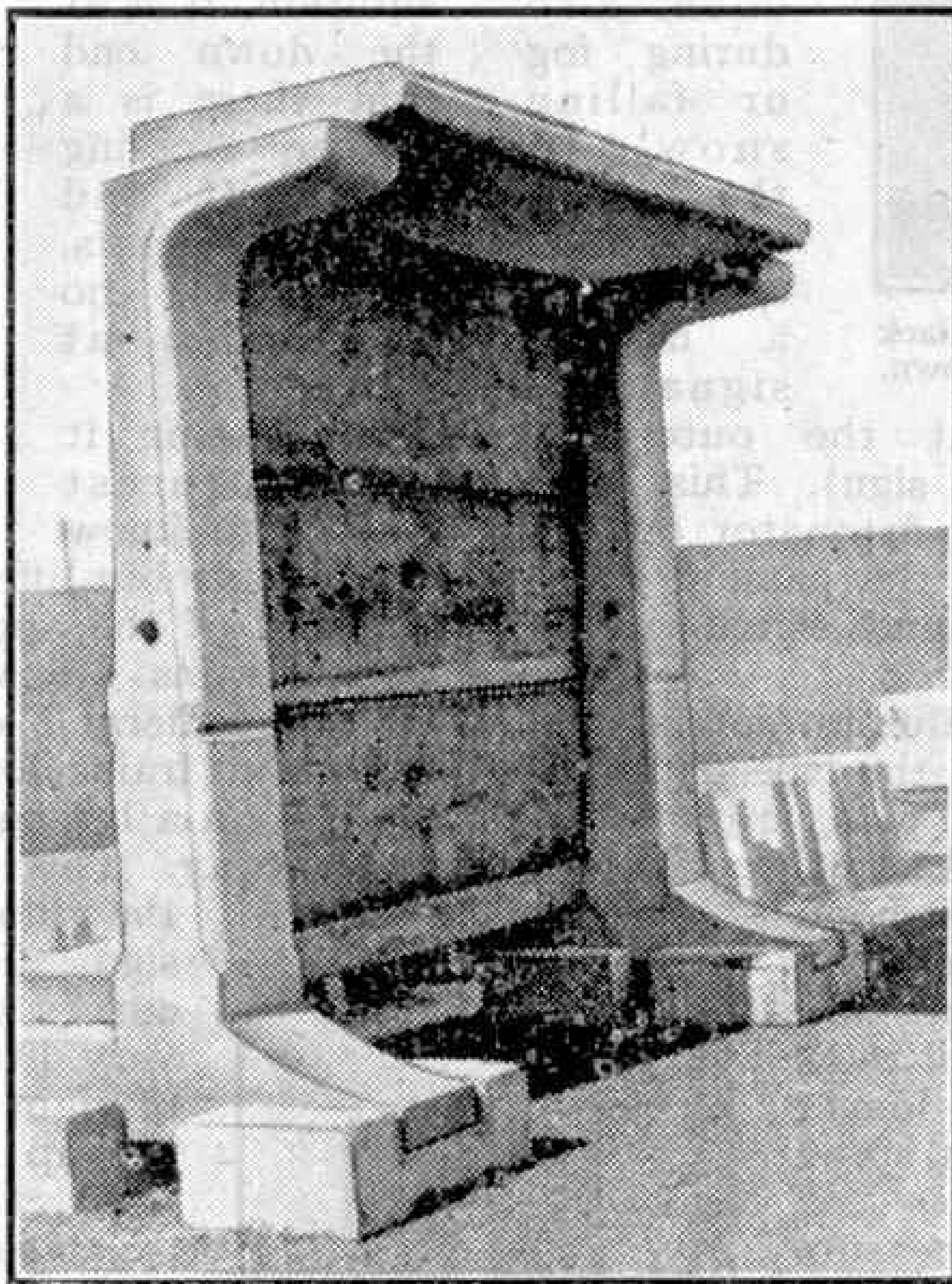
How the pre-cast concrete platform units fit.
