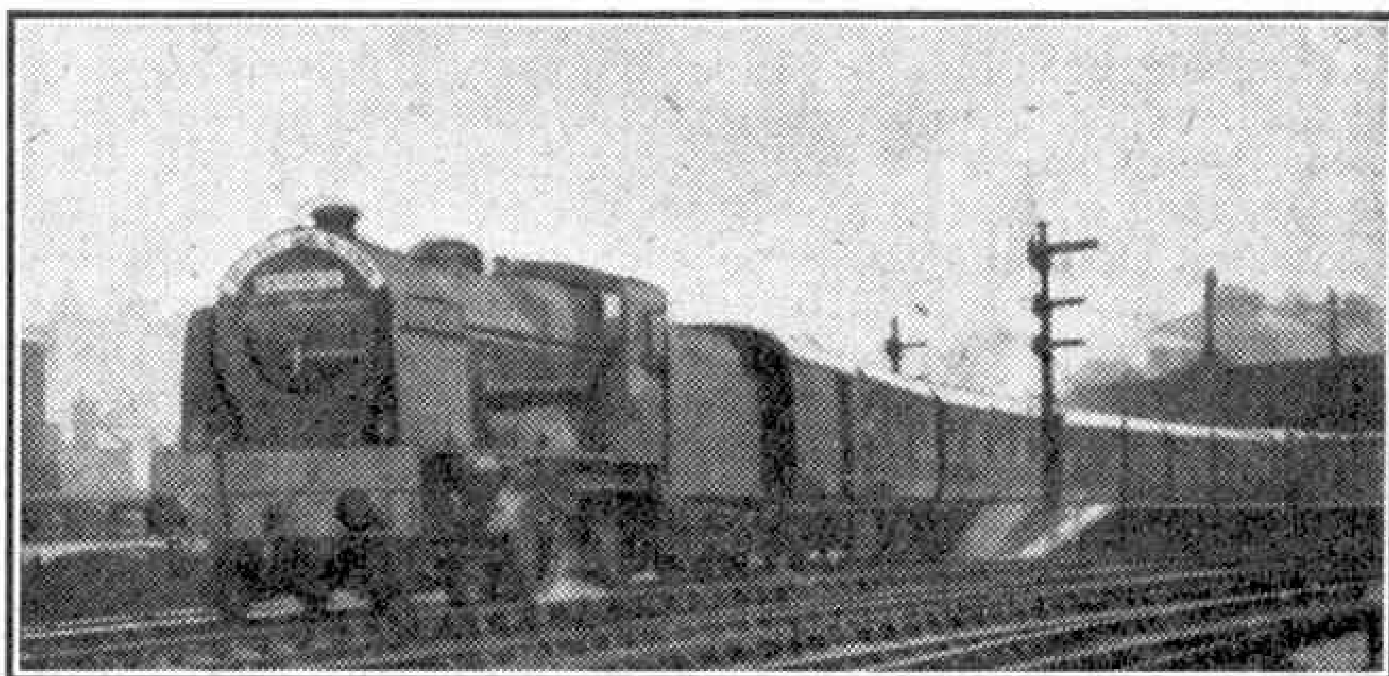
The Belfast-Cork "Enterprise" leaving Belfast on its first trip. The engine is G.N.R. 3-cylinder simple 4-4-0 No. 206 "Liffey."
