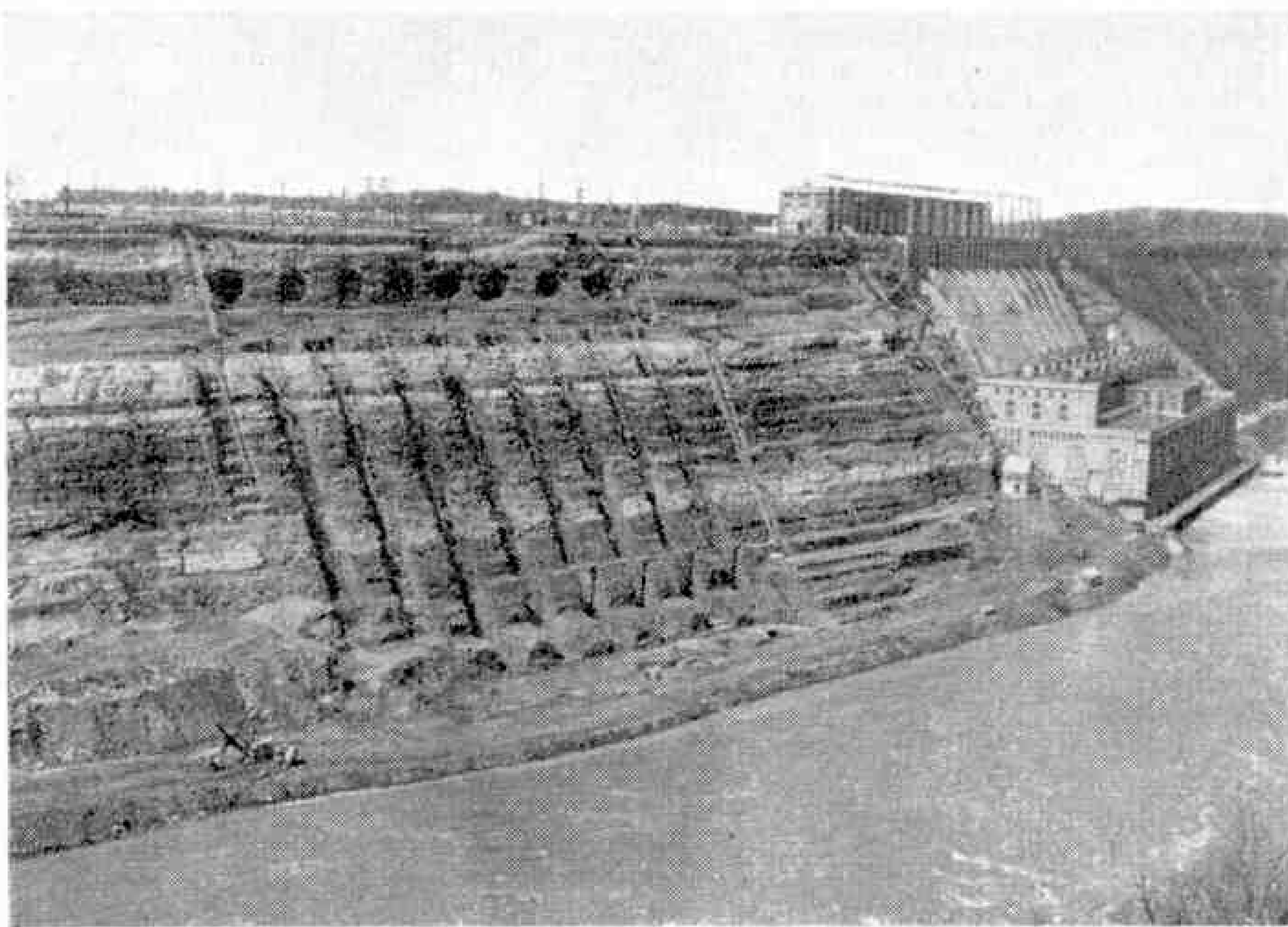
Where the new power station on the Canadian side of the Niagara River will be built. In this picture the excavation work is seen in progress, and the existing power station also is visible.
