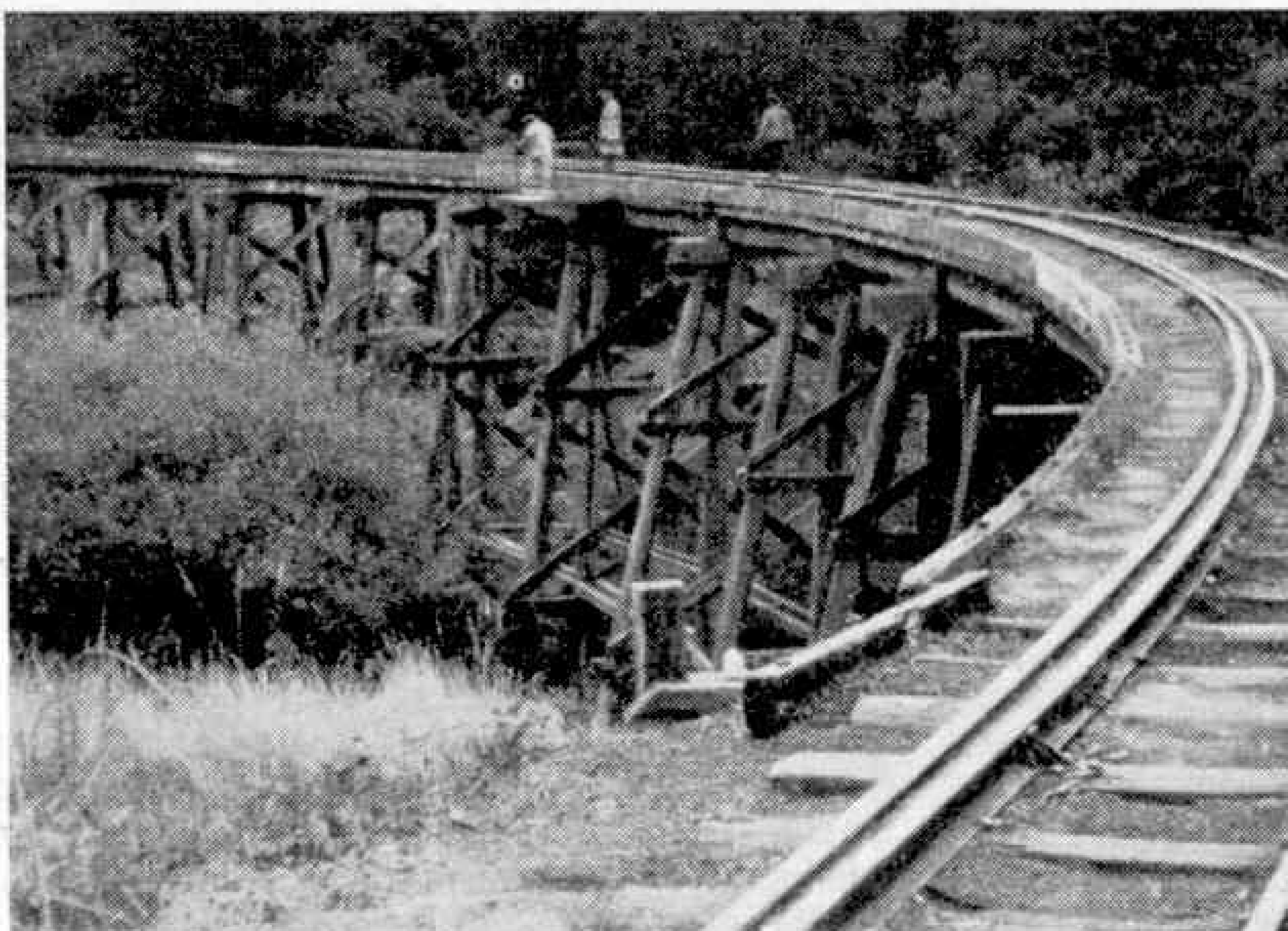
Horseshoe Bridge, Selby, a long trestle structure.
