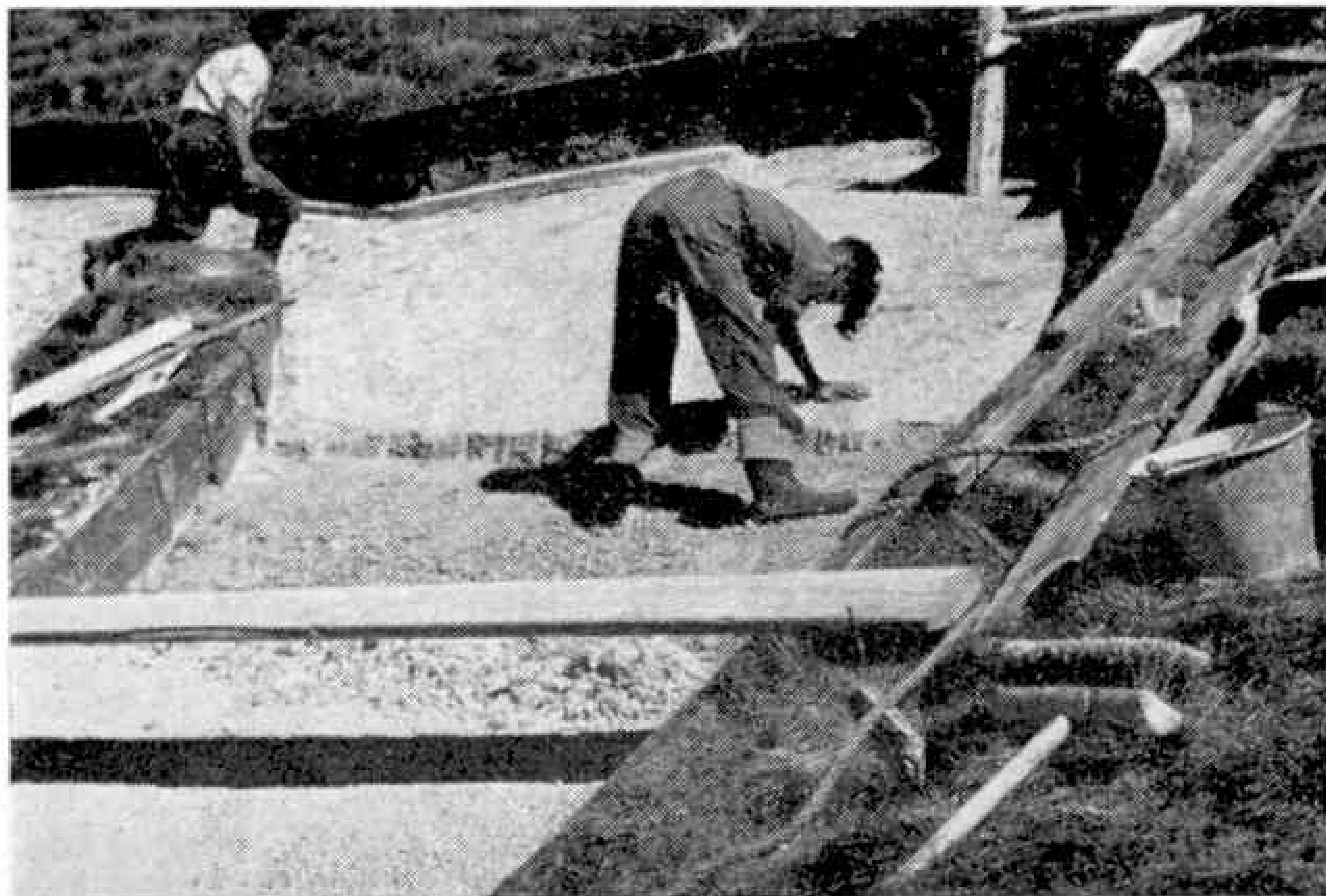
Replacing the tail of the Westbury White Horse by a mixture of cement, chalk and gravel. Photograph by Geoffrey N. Wright, Limpley Stoke.
