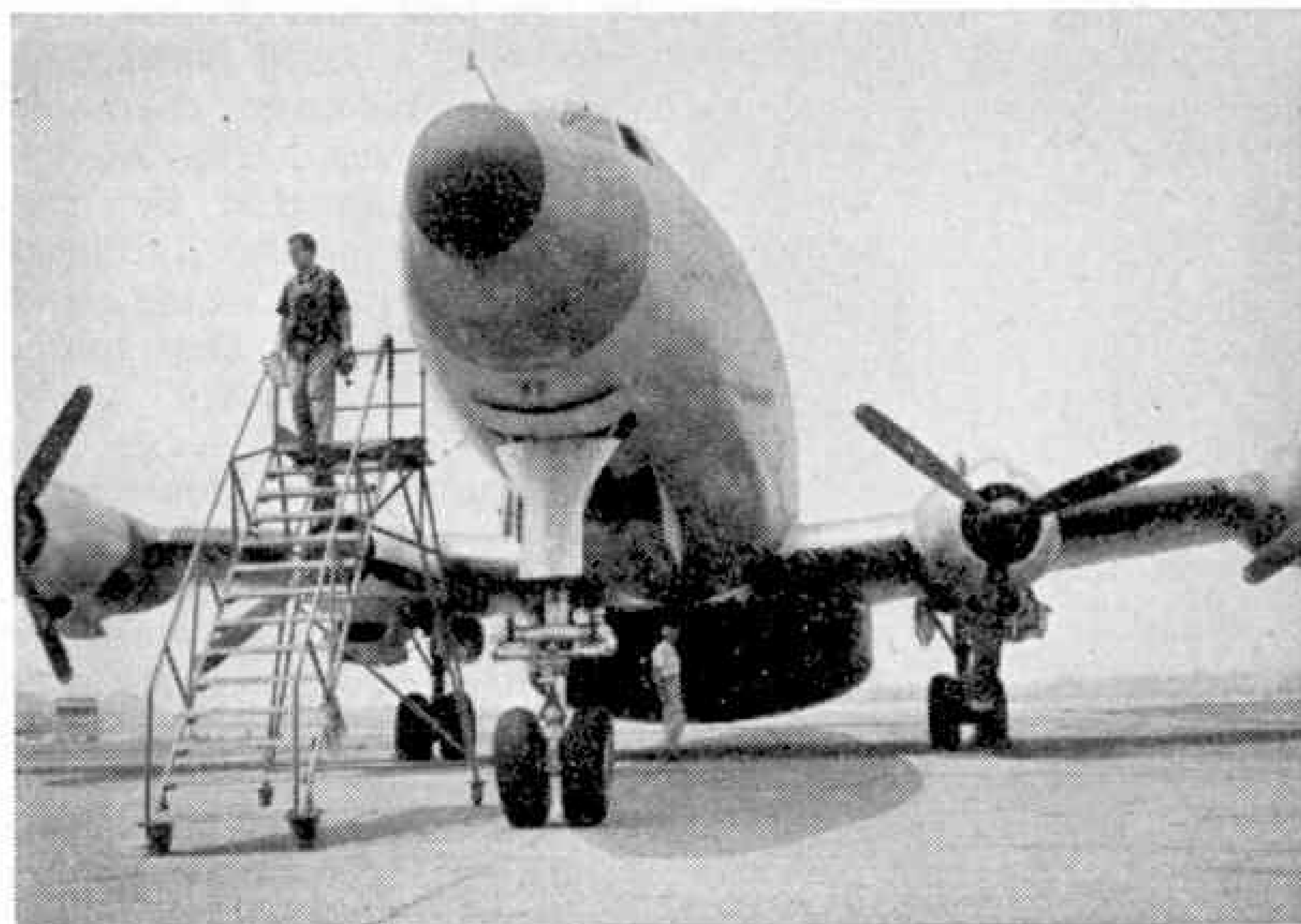
Ground view of the RC-121C. The 8ft. high hump on the back, the huge bulge underneath and the elongated nose house radar antennæ.
