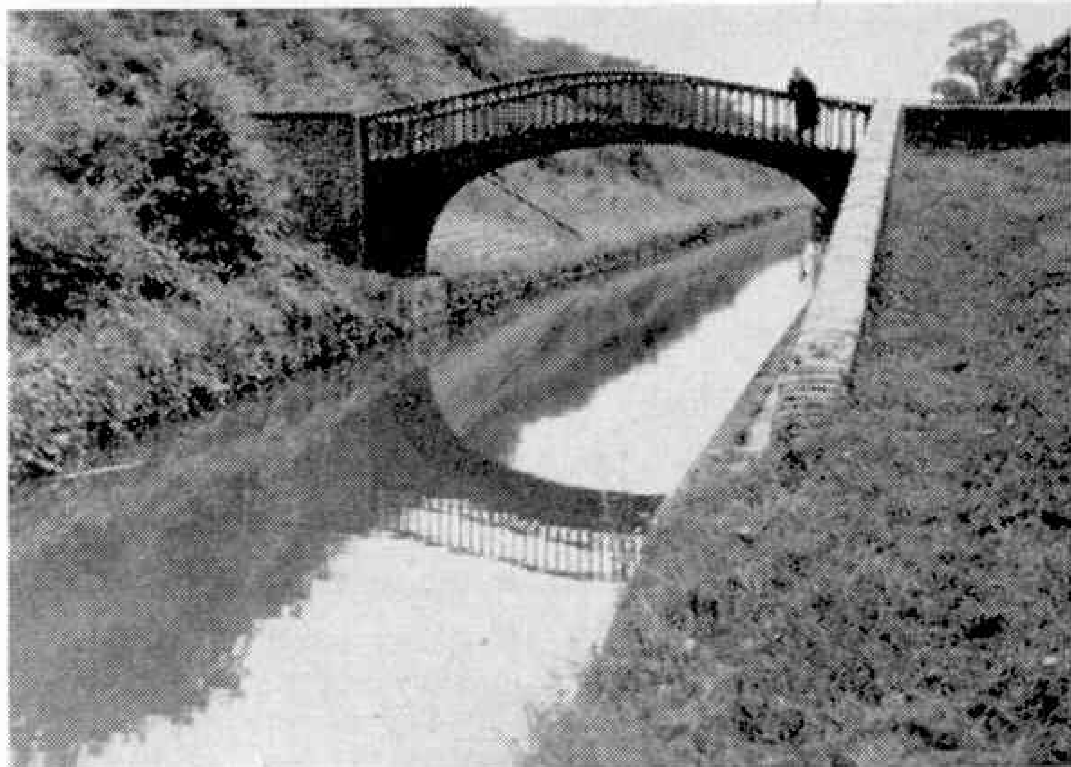
The Oxford Canal at Fenny Compton is in a deep cutting formed by opening out the tunnel originally built there.
