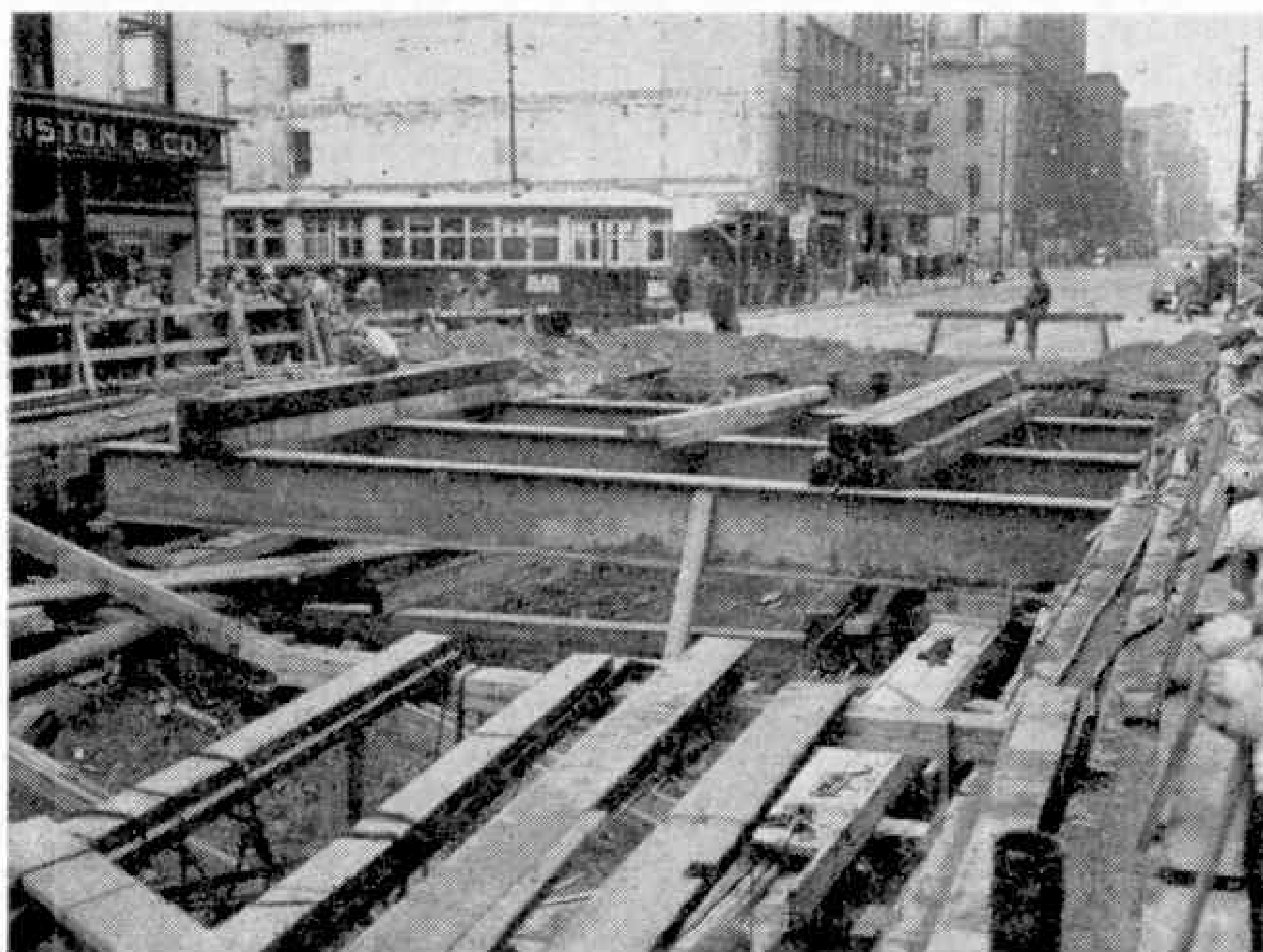
Early stage of excavation of a block of Yonge Street. Steel beams are being put in position to support a temporary wooden street surface, while excavation continues below.
