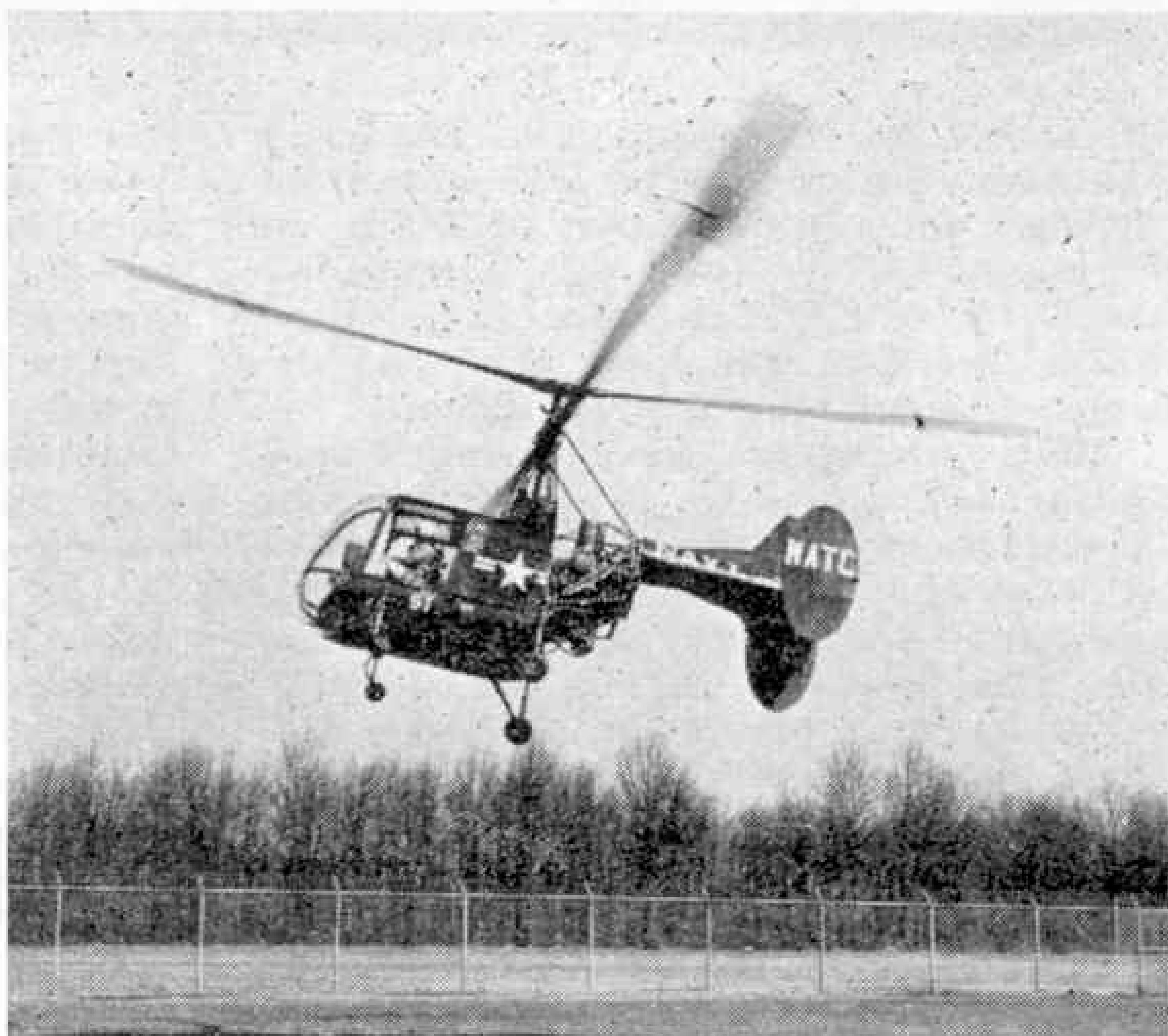
The Kaman HTK-1, shown above, is the world's first twin-turborotor helicopter, and a joint U.S. Army-Navy project. U.S. Department of Defense photograph.
