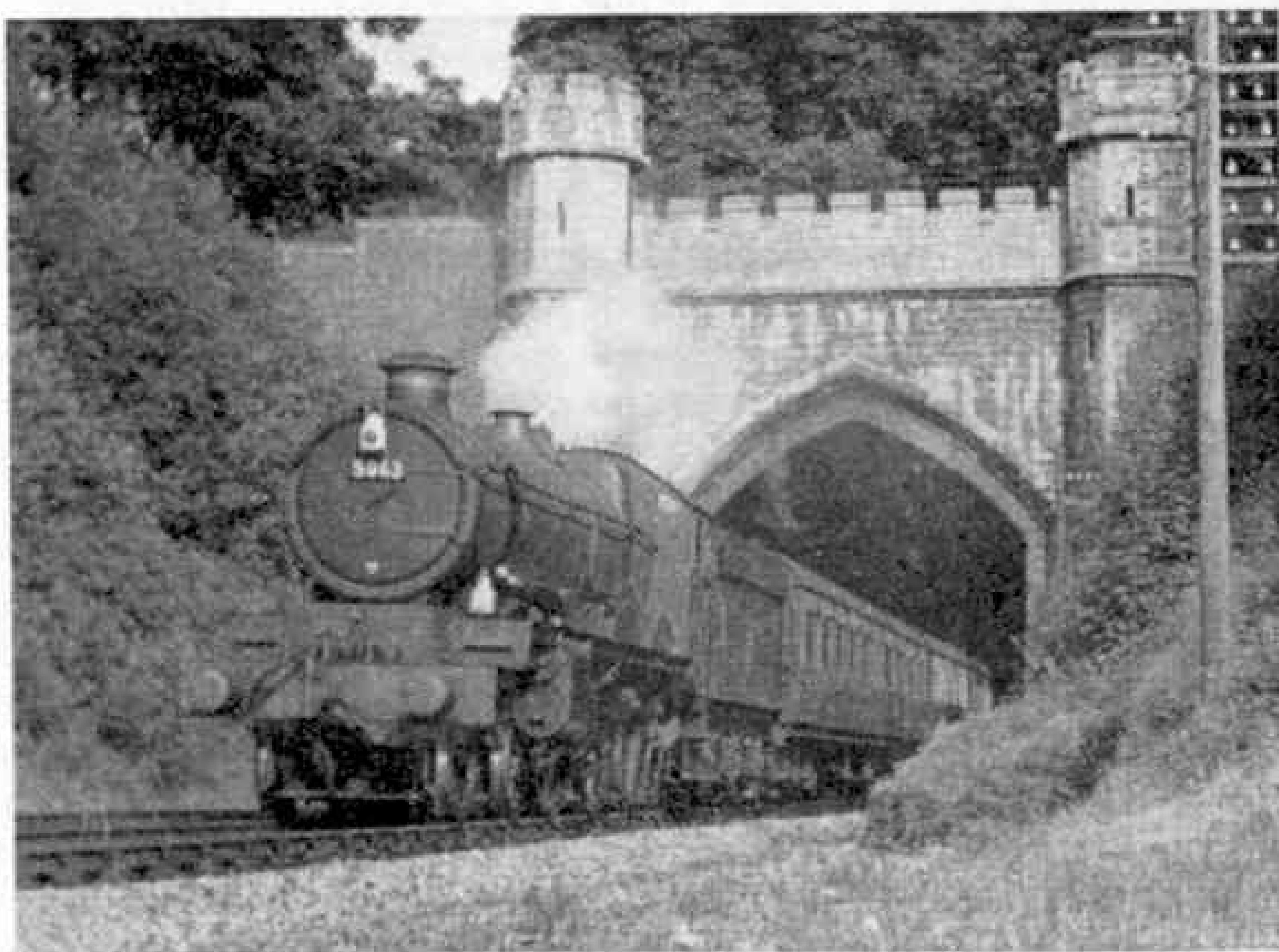
No. 5063 "Earl Baldwin," of the Castle class, emerges from one of the picturesque ends of Twerton Tunnel. Photograph by R. E. Toop.
