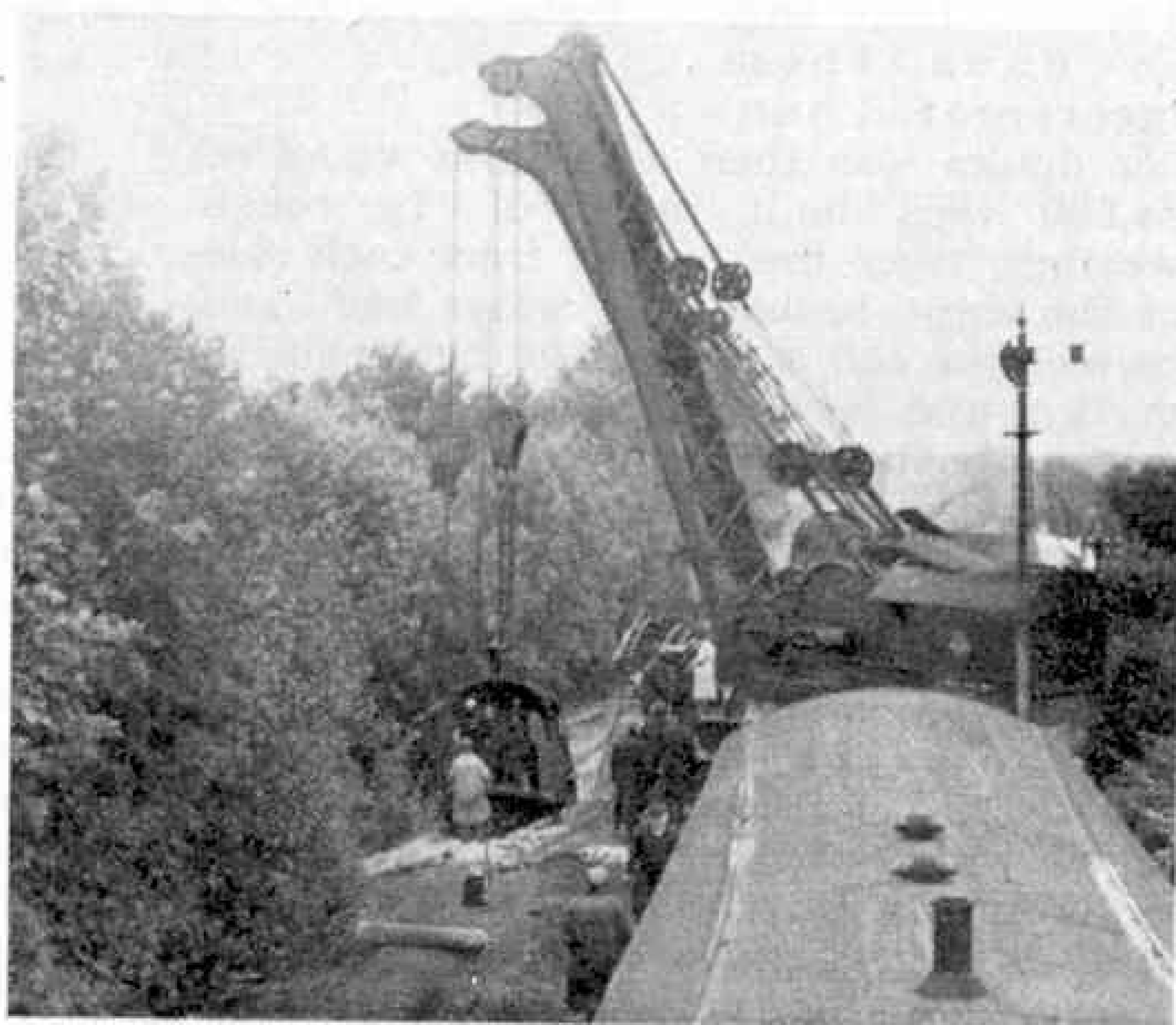
Two 36-ton cranes preparing to lift the engine, as seen from the roof of the breakdown train.
