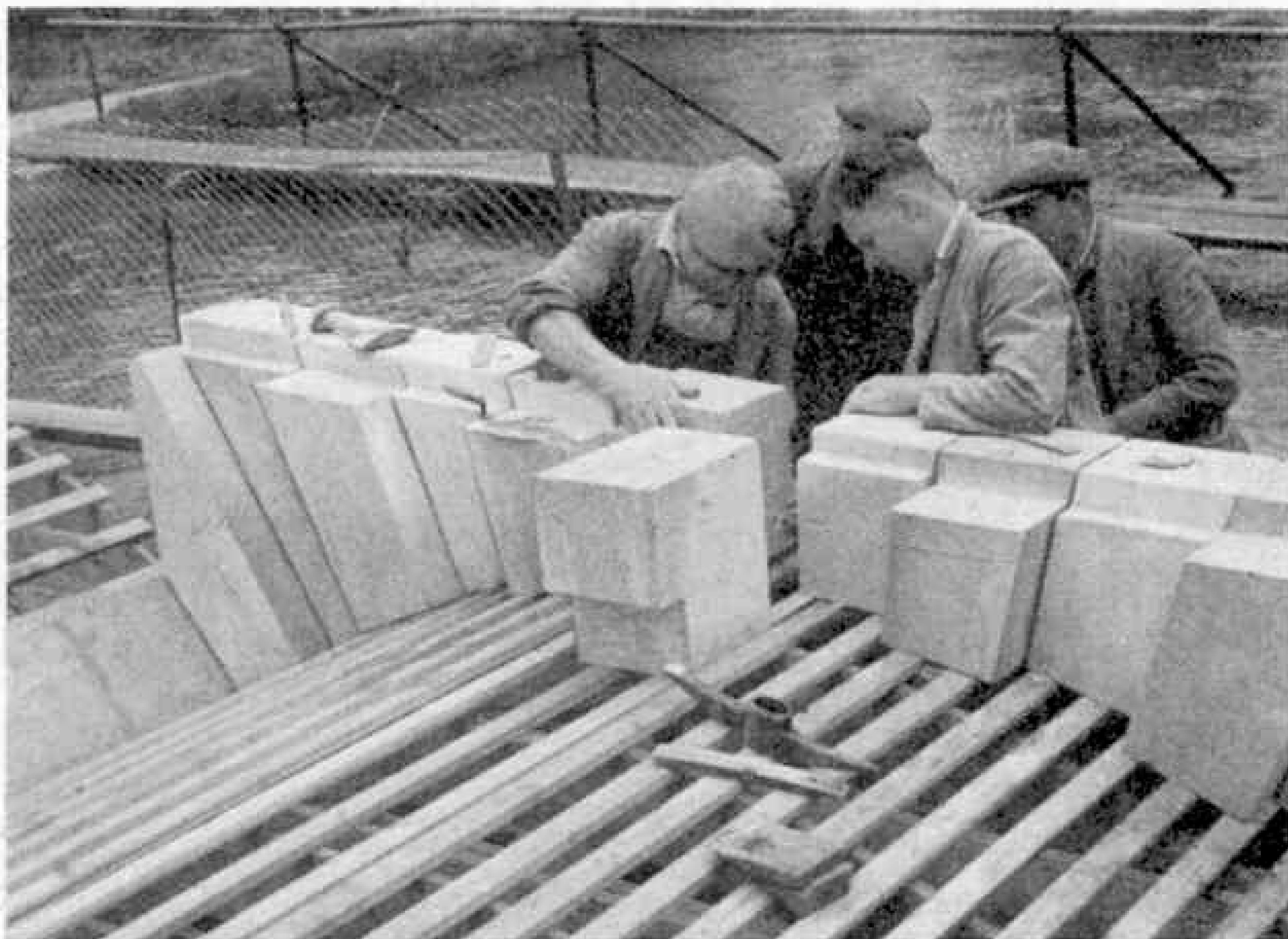
The building of a masonry arch bridge at Bourton-on-the-Water, Gloucestershire, is shown in these pictures. In the lower one the keystone of the arch is about to be placed in position. Photographs by W. S. Garth.
