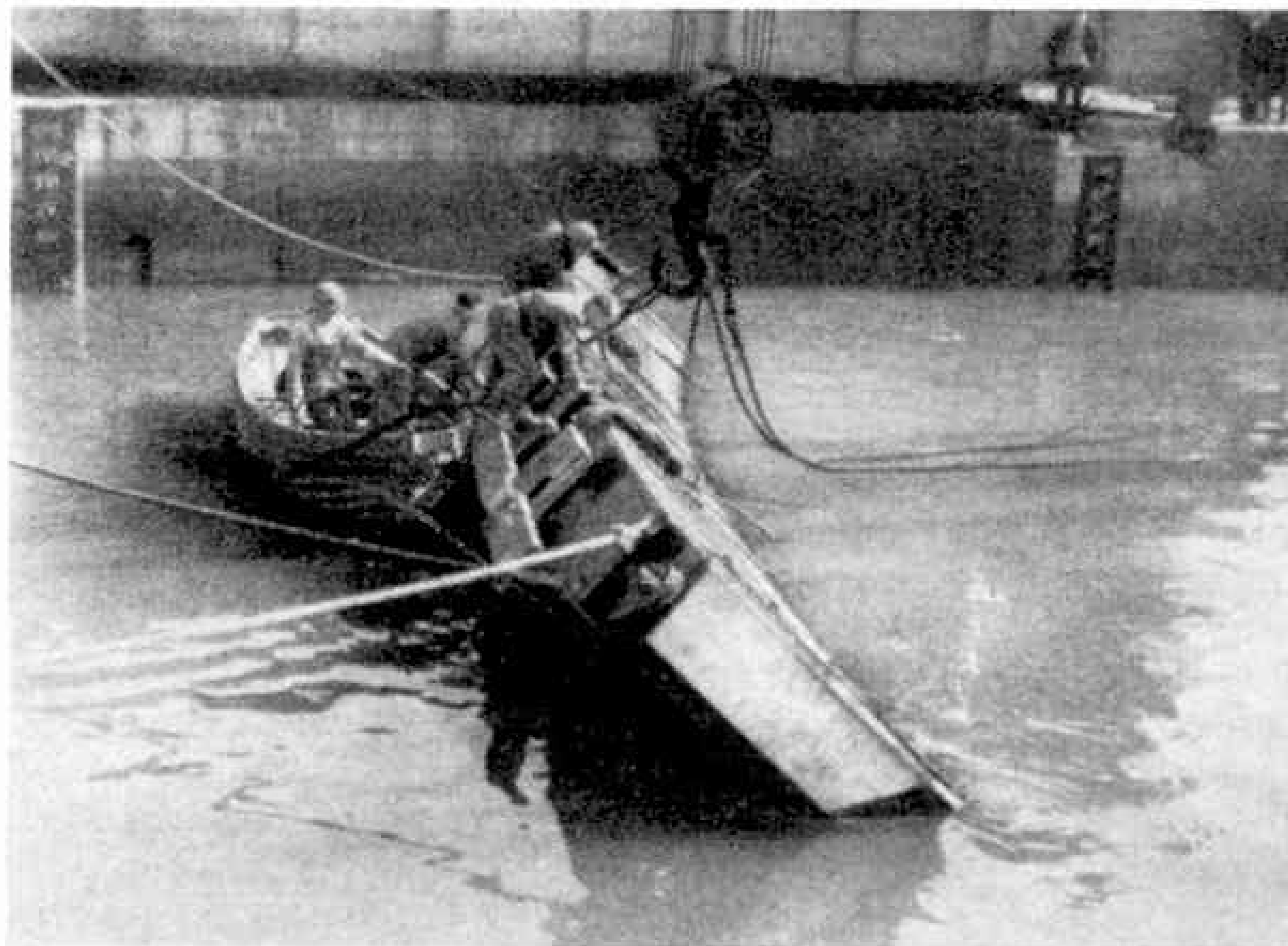
A leaf of the gates of one of the Docks of the Dover Harbour Board being re-positioned.
