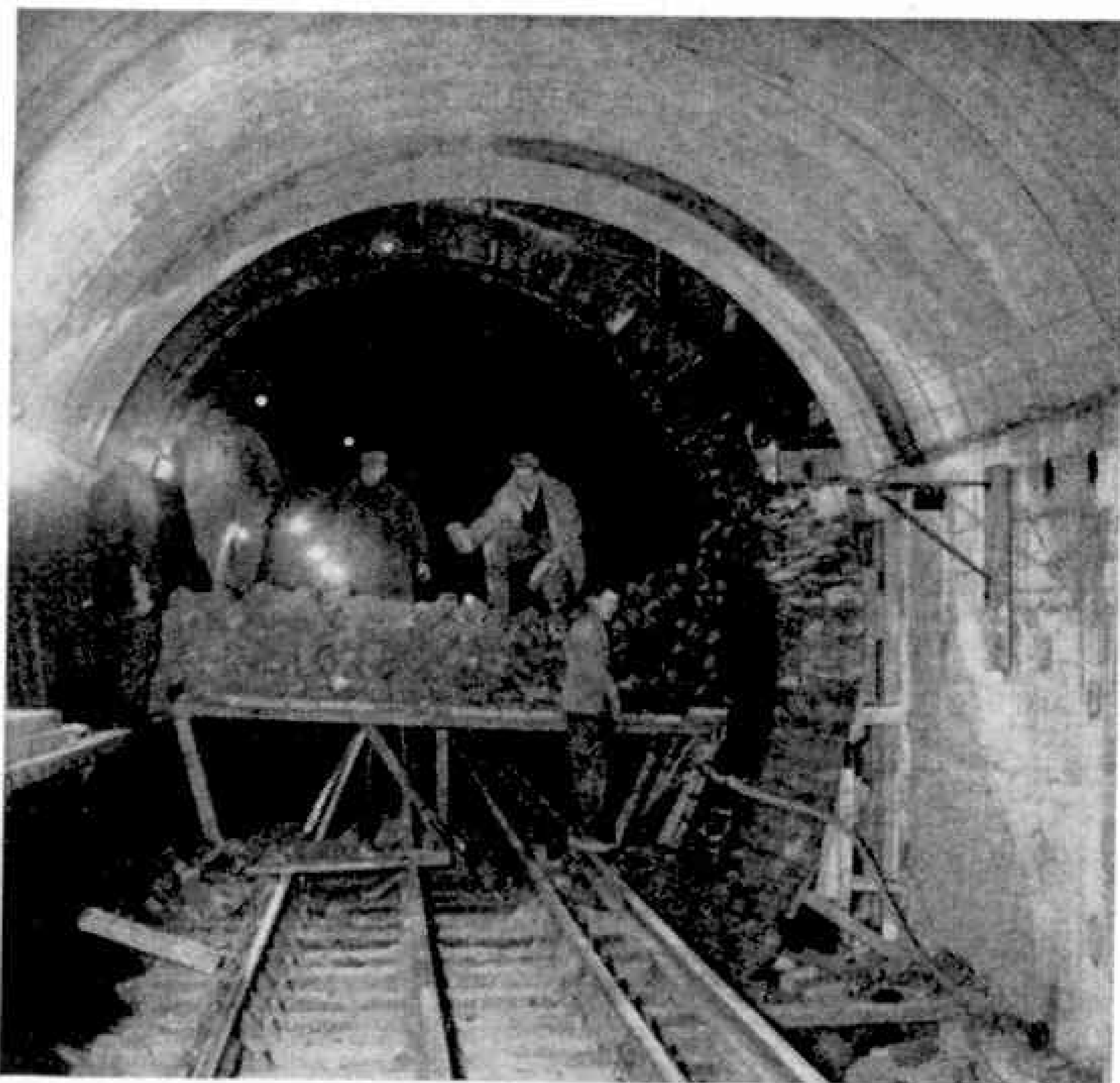
Renewing an old tunnel near Swiss Cottage on the Metropolitan Line. The section of old brickwork that has been broken down lies on the working stage ready for removal.
