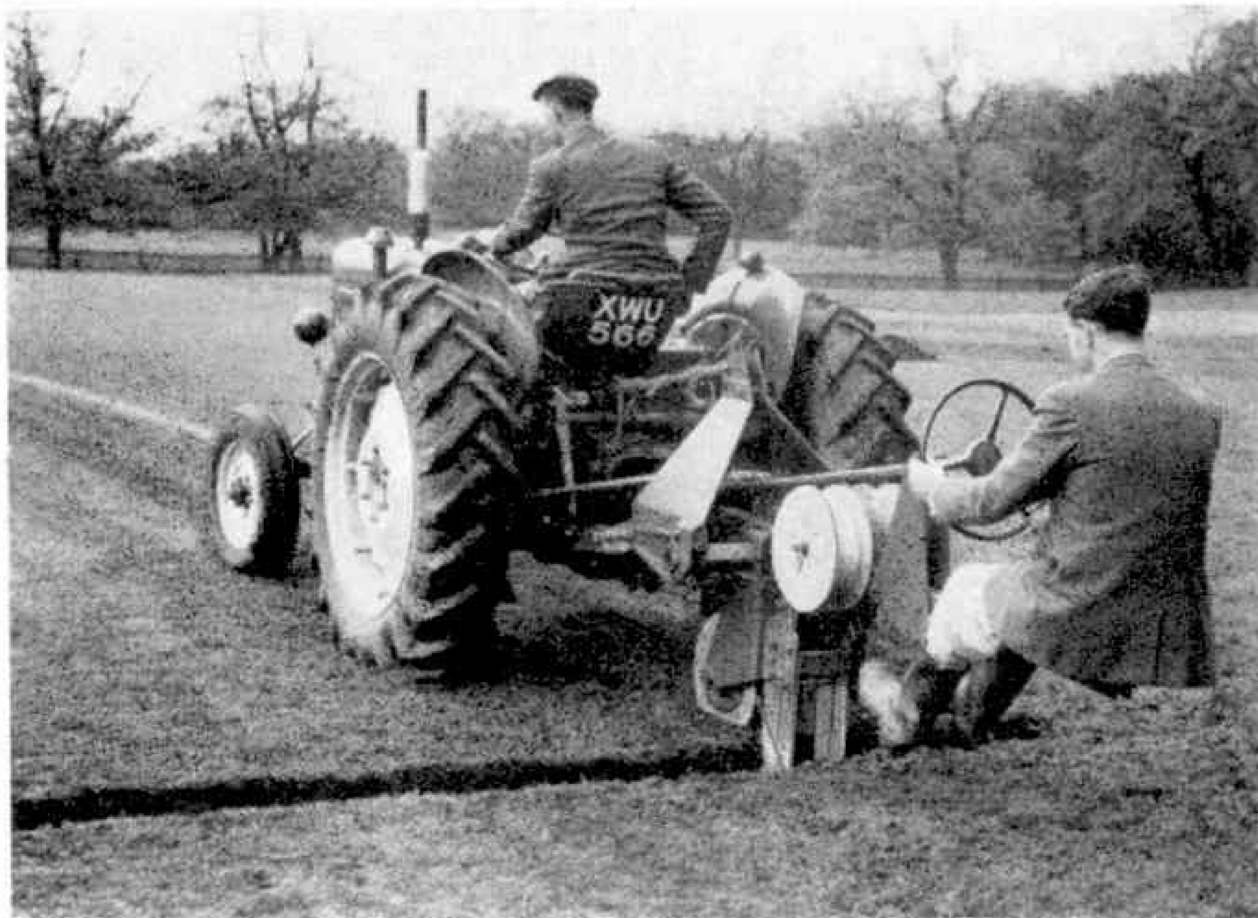
The David Brown Albion underground cable-laying machine at work on a sports ground. Photographs by courtesy of David Brown Tractor Division.
