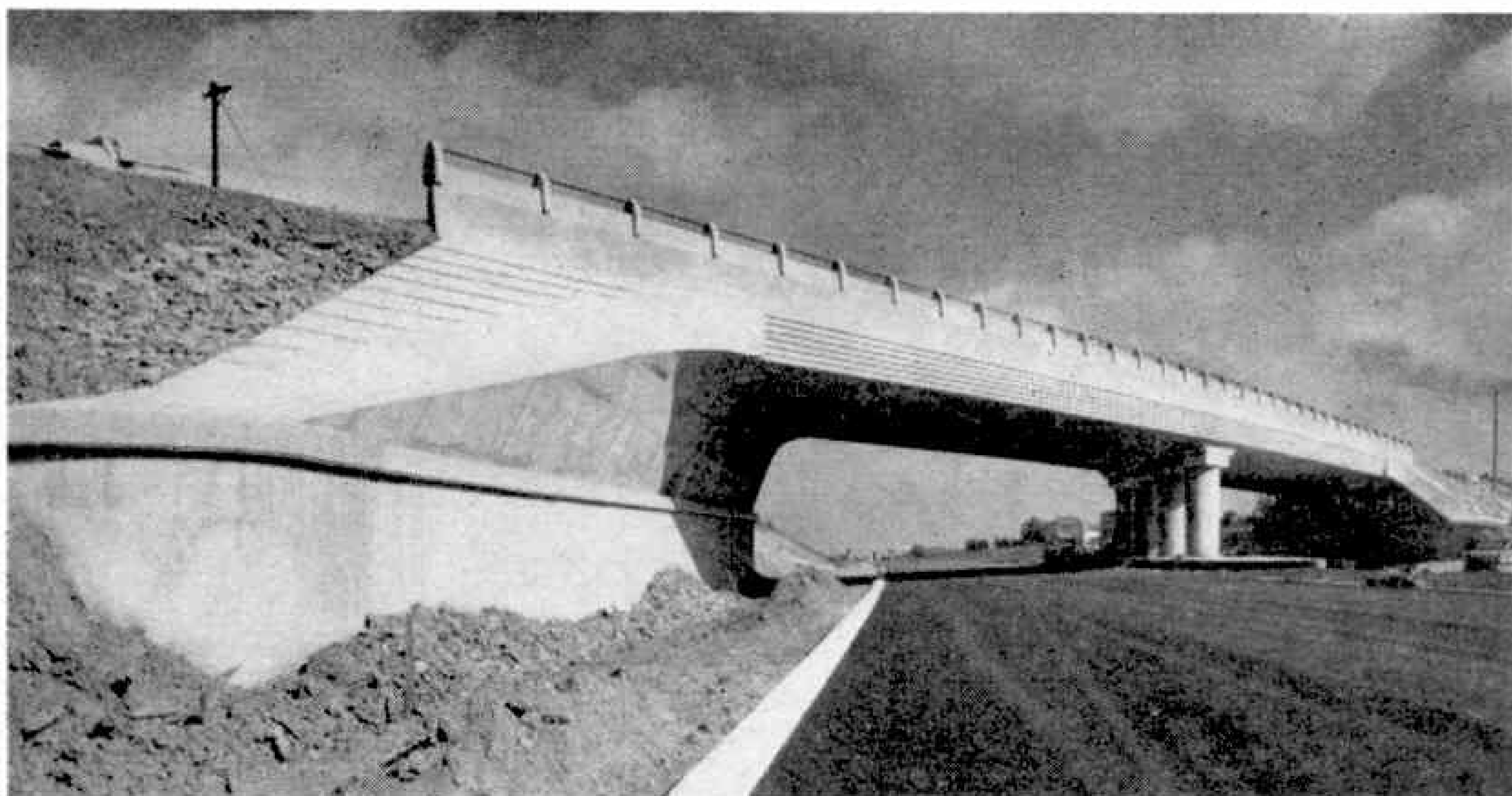
This fine two-arch bridge on Britain's motorway is "Structure 62", near Hanslope, Bucks.
