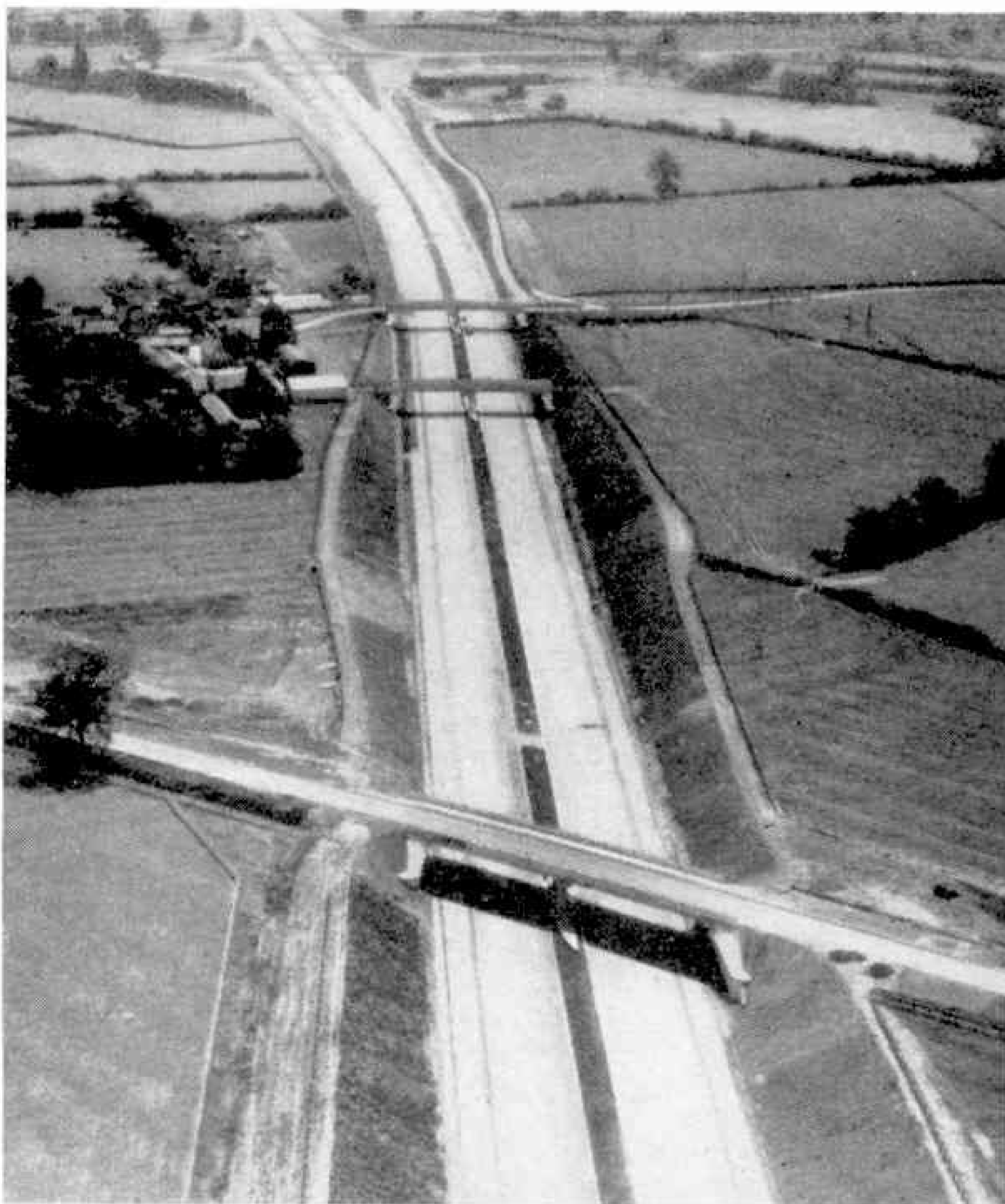
Another section of the motorway.
