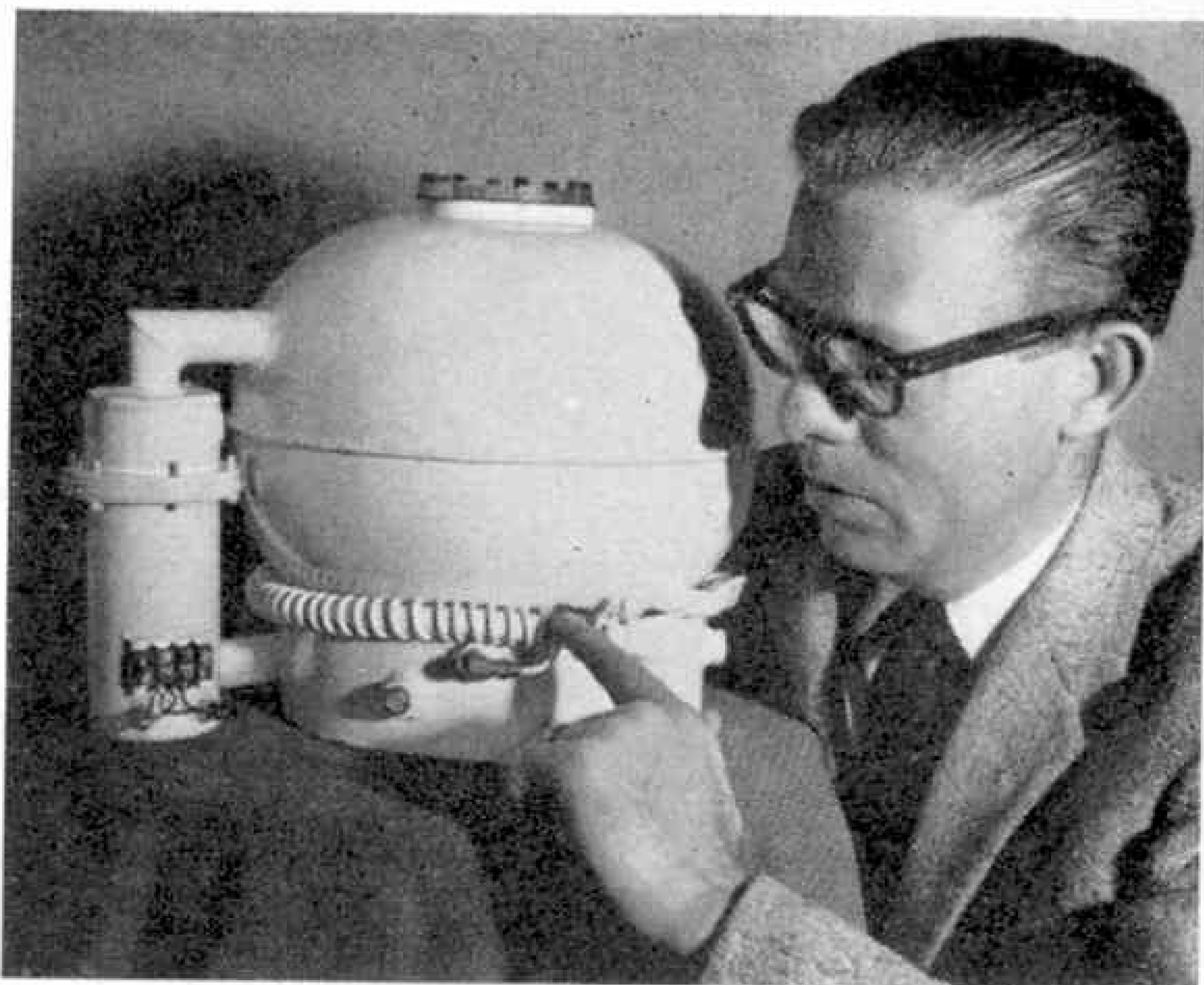
The engineer in charge of the development of the mouse house described on these pages points to a copper tube around the animal space capsule which is used to cool the oxygen. Photograph by courtesy of the Garrett Corporation.
