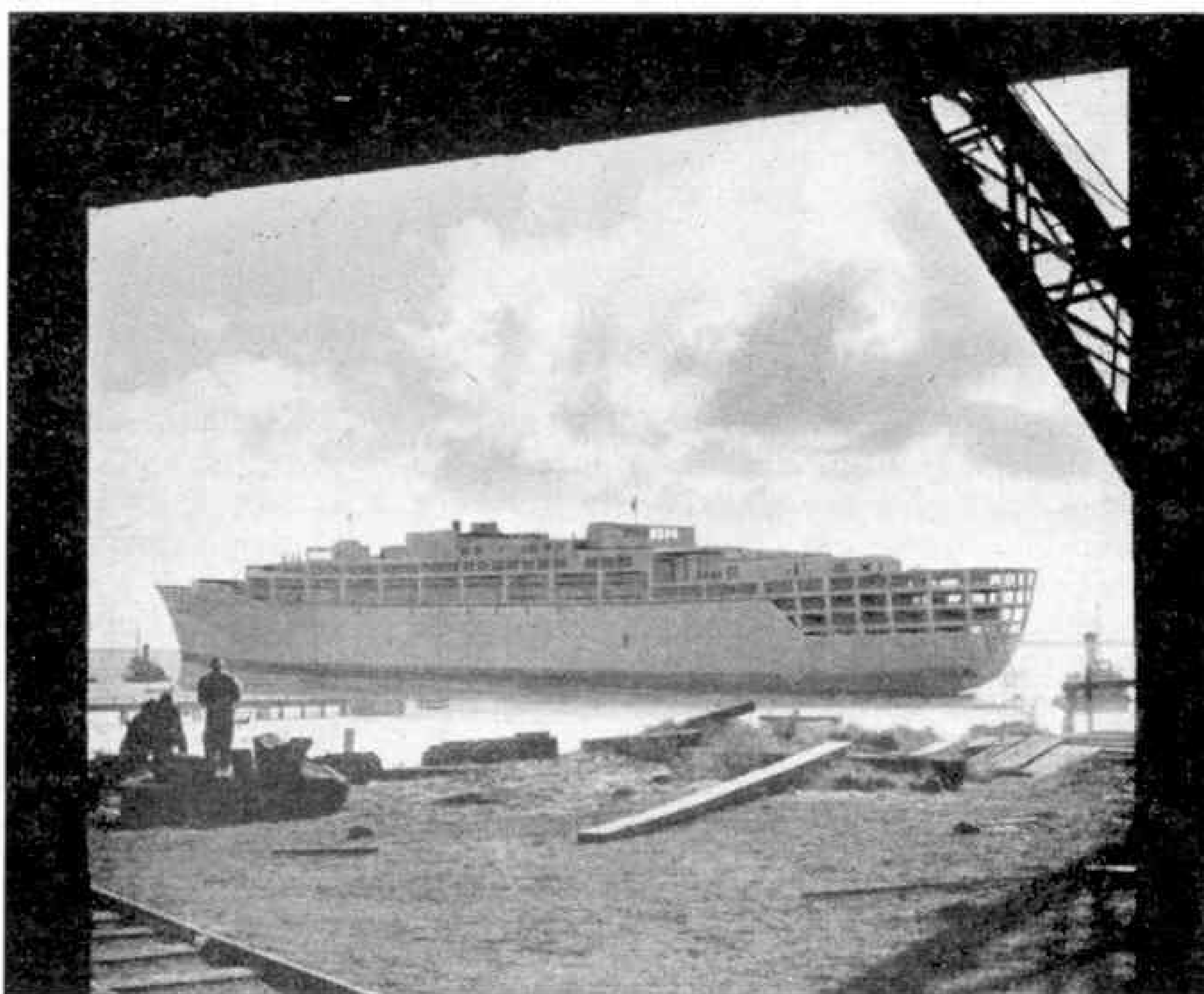
" Oriana " is towed to the fitting-out berth after launching.
