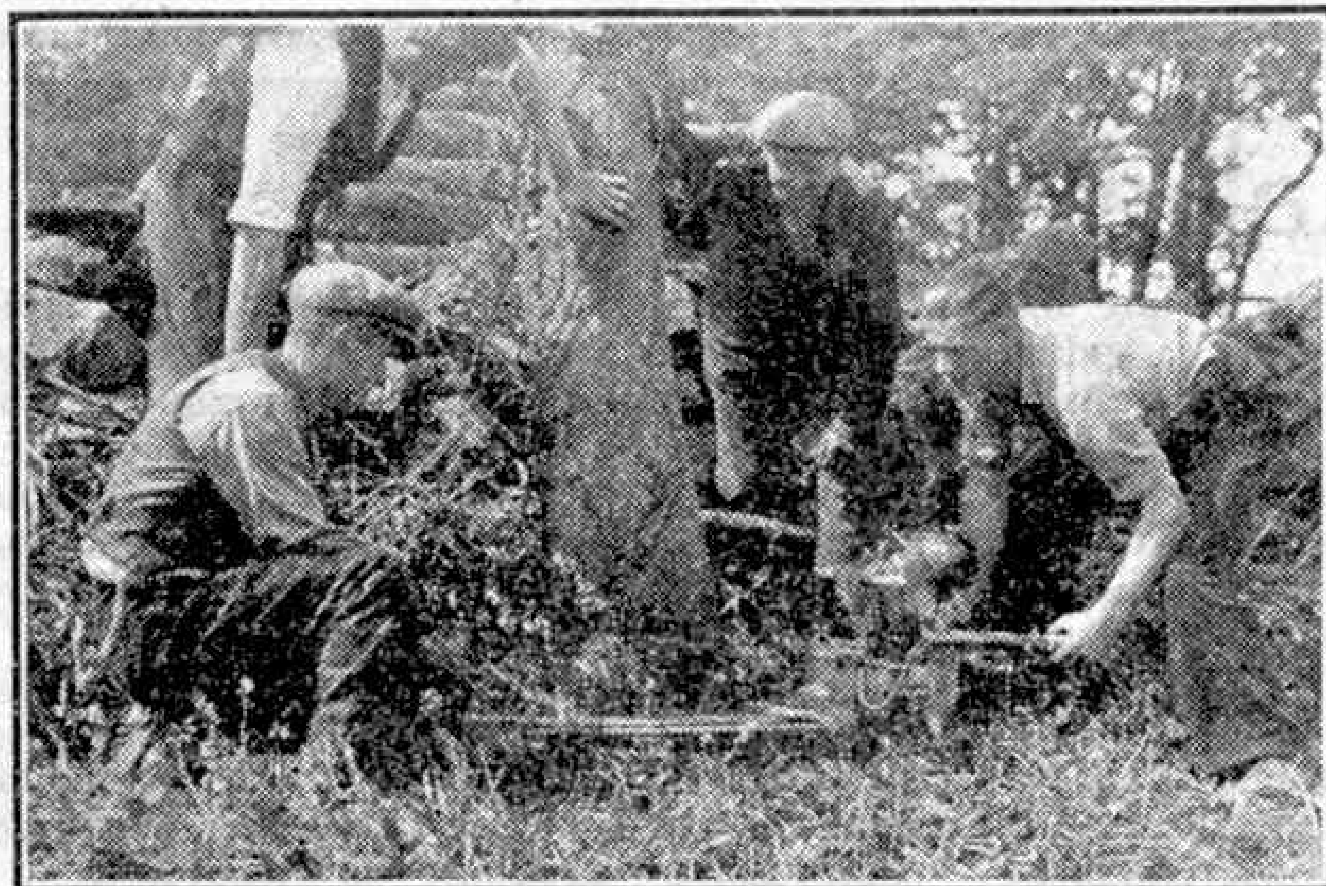
A power driven saw in operation. With its 1\frac{1}{2} h.p. motor this can fell a large tree in 1\frac{1}{2} min.
