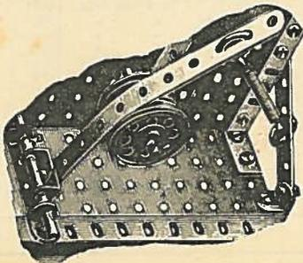
C—Spring controlled Band Friction Brake
