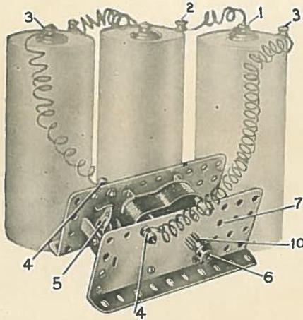
one-way motor in motion. Insulated copper bell wire is recommended for making the connections and can be obtained at any electrical supply store.
